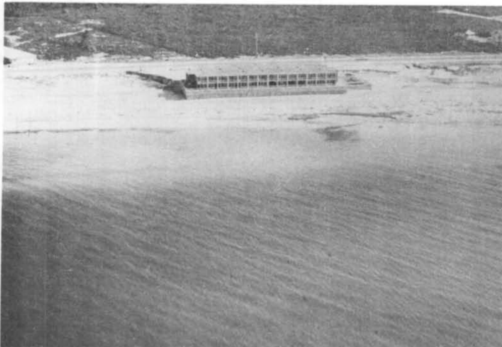
Figure 4. Effects on an Adjacent Beach Caused by a Vertical Faced Seawall (Courtesy of Professor Byron Spangler)
