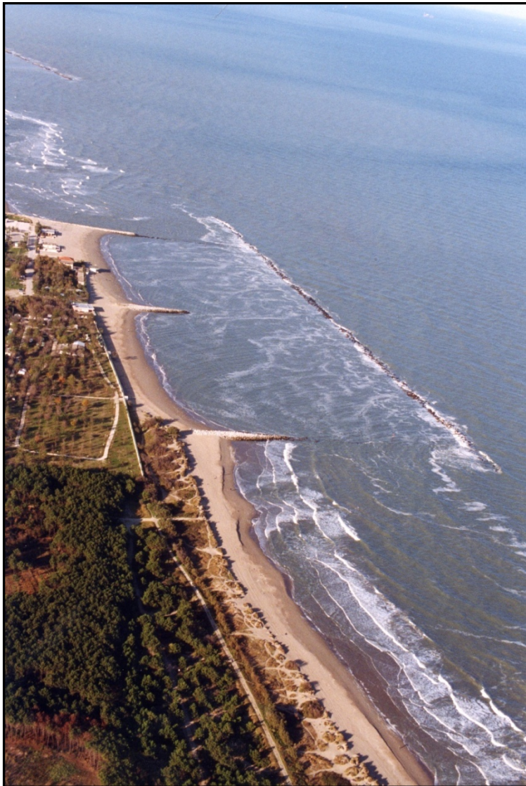
Fig. 4.2. Aerial view of the shoreline and the coastal-defence system at Lido di Dante (Ravenna, Italy). Photo by Giorgio Benelli, published with permission.
