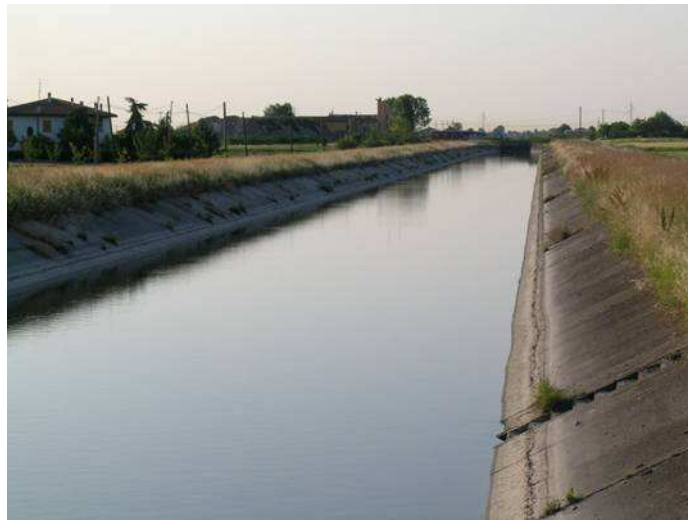
Figure 8 – View of the irrigation canal Canale Emiliano Romagnolo (CER).
