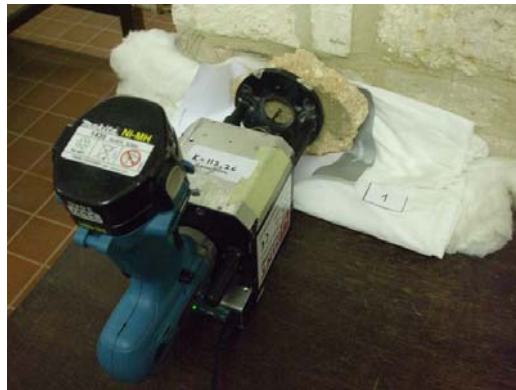
Fig.20 Molab drilling tests on mortar. The driller.
