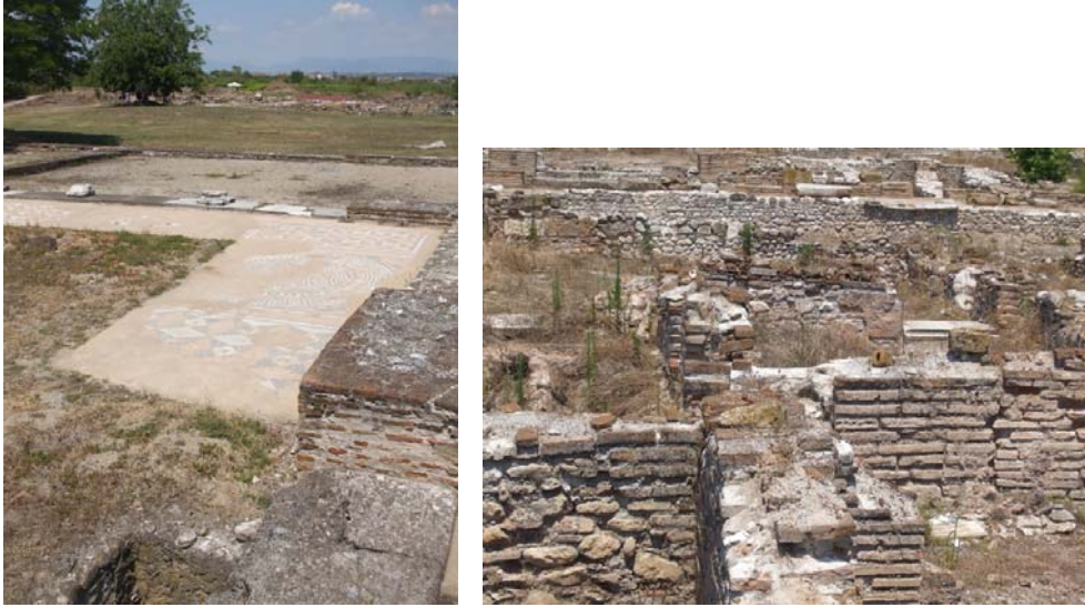
Fig.102-103 Views of the site showing the walls in opus incertum , opus mixtum .
