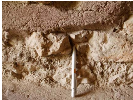
Fig.90 Example of structural mortars without the presence of brick fragments as aggregates, from walls in open air conditions. Fig.91 Detail of walls preserved in the covered area of the site (at the top of the picture the red line marker).
