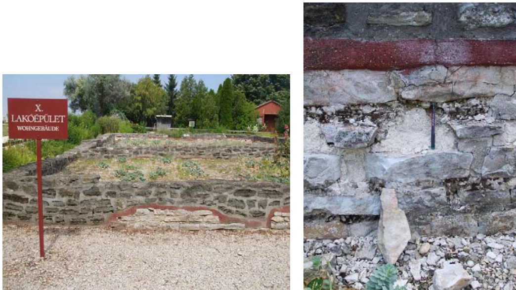
Fig.87 A view of the entrance of the site and the reconstructed walls. In the second picture a detail of the lowest part of the wall, supposed to be original. The red line (cement) is the marker of the replacing and restoring intervention.
