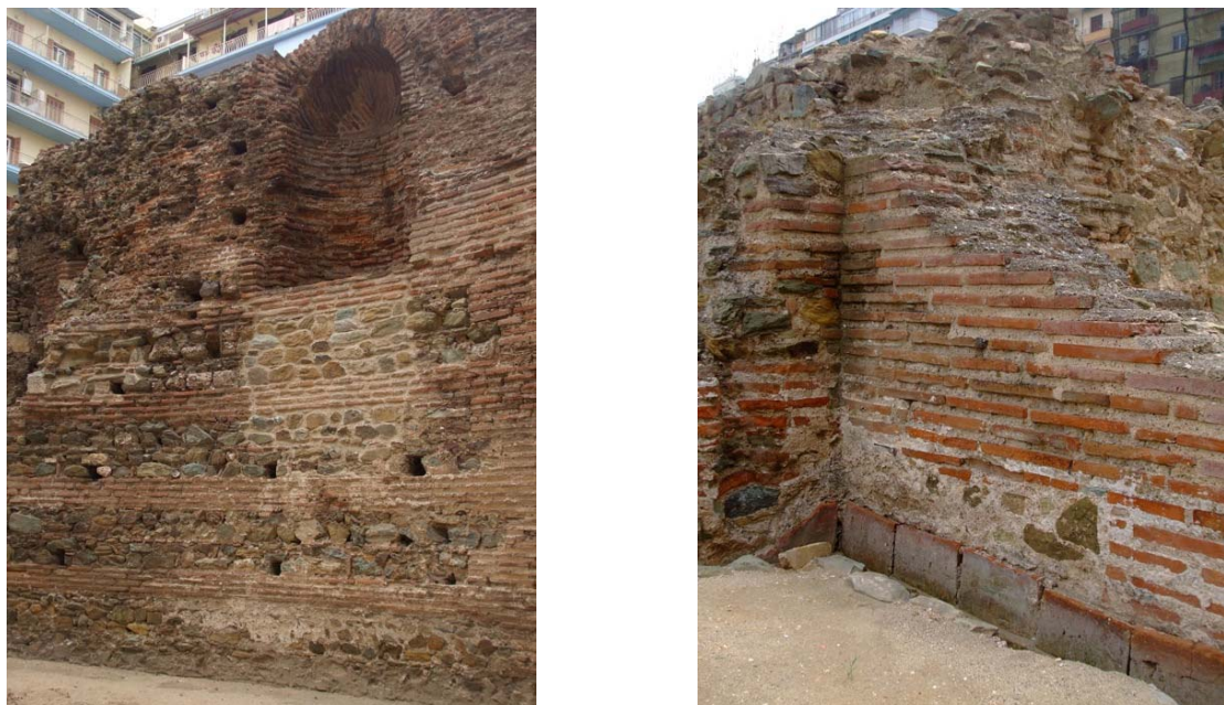
Fig.94-95 On the left a detail of a wall of the Basilica in opus mixtum (Galerius Palace in Thessaloniki) on the right bricks wall in opus signinum (lime based mortar with brick fragments as aggregates, cocciopesto )
