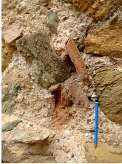
Fig.110-111 Details of opus caementicium : on the left detail from Dion, on the right detail from the Galerius Palace.
