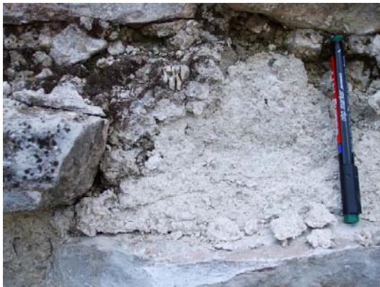
Fig.90 Example of structural mortars without the presence of brick fragments as aggregates, from walls in open air conditions. Fig.91 Detail of walls preserved in the covered area of the site (at the top of the picture the red line marker).
