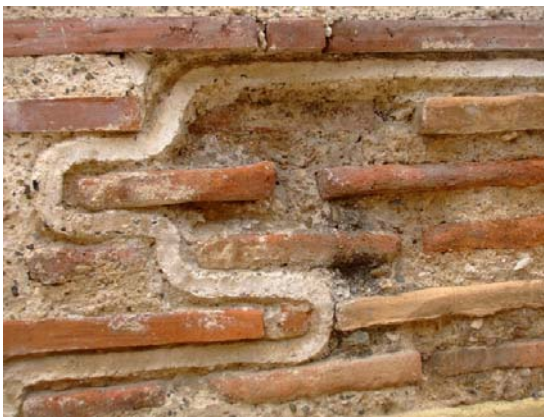
Fig.98-99 Details of the mortar strip used as marker of the reconstructive intervention (Galerius Palace in Thessaloniki)
