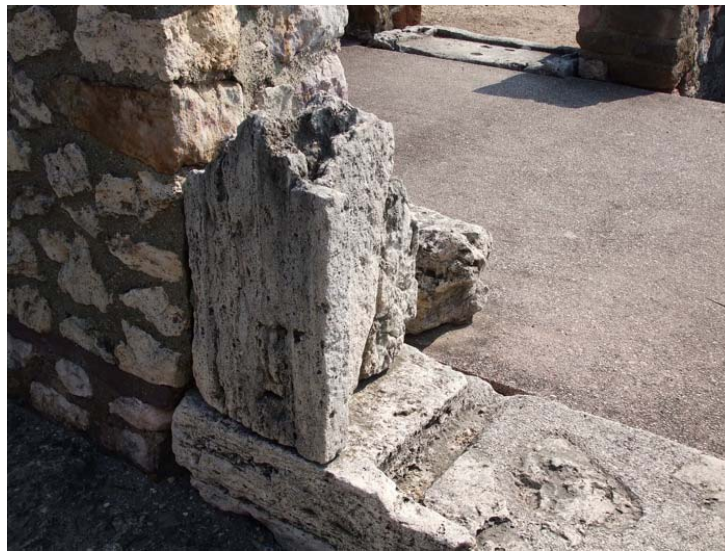
Fig.82 The use of travertine for structural elements.
