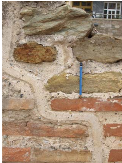
Fig.98-99 Details of the mortar strip used as marker of the reconstructive intervention (Galerius Palace in Thessaloniki)
