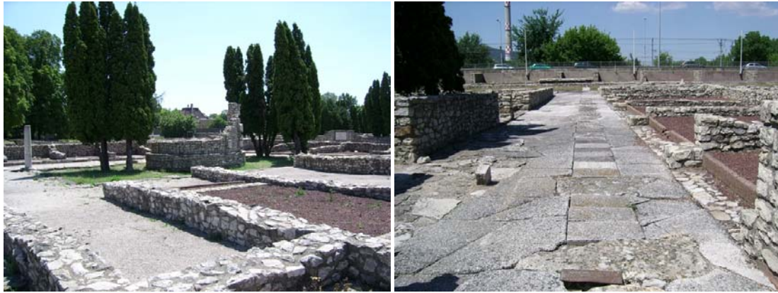
Fig.80-81 Two different views of the site. In the first the reconstructed walls are visible, in the second the partially reconstructed Roman road.
