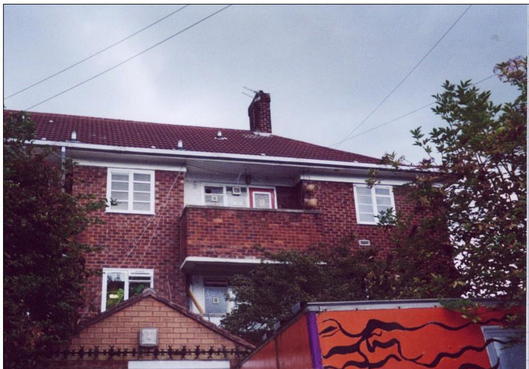
Figure 4-3: View of maisonettes showing computer data cables strung across street (top right hand of photo) and from top balcony to lower flats (centre)
