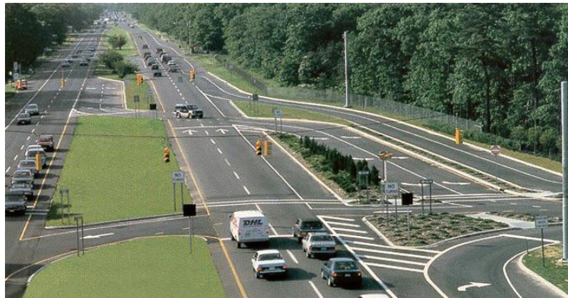
Figure 4: Dowling College, New York: A prototype CFI was built at a T intersection http://teexwebtest.tamu.edu/eu/documents/04_01-02.pdf
