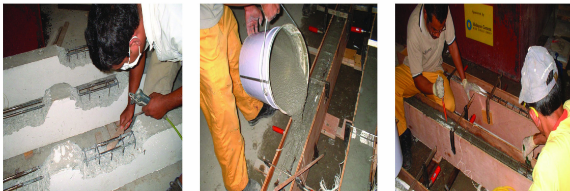
Plate 1: a) Surface Preparation b) Application of Sika Microcrete 2000 to Beam Surface and c) Sika MonoTop R40 on wet surface
