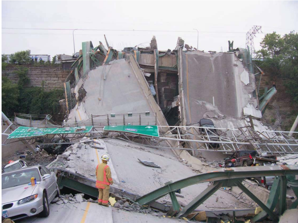
Figure 1-1. Scene of the collapse, the Interstate 35W Bridge over the Mississippi River in Minneapolis, Minnesota, 2007 [145]
