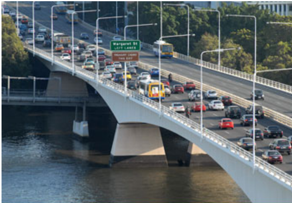
Figure 1-2. The Captain Cook Bridge over Brisbane River (Courtesy of Tim Marsden)
