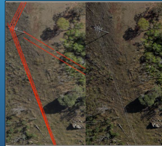
Automated inspection of power lines. Photo taken from a UAS with automated power line detection algorithm (ARCAA and CRC-SI)
