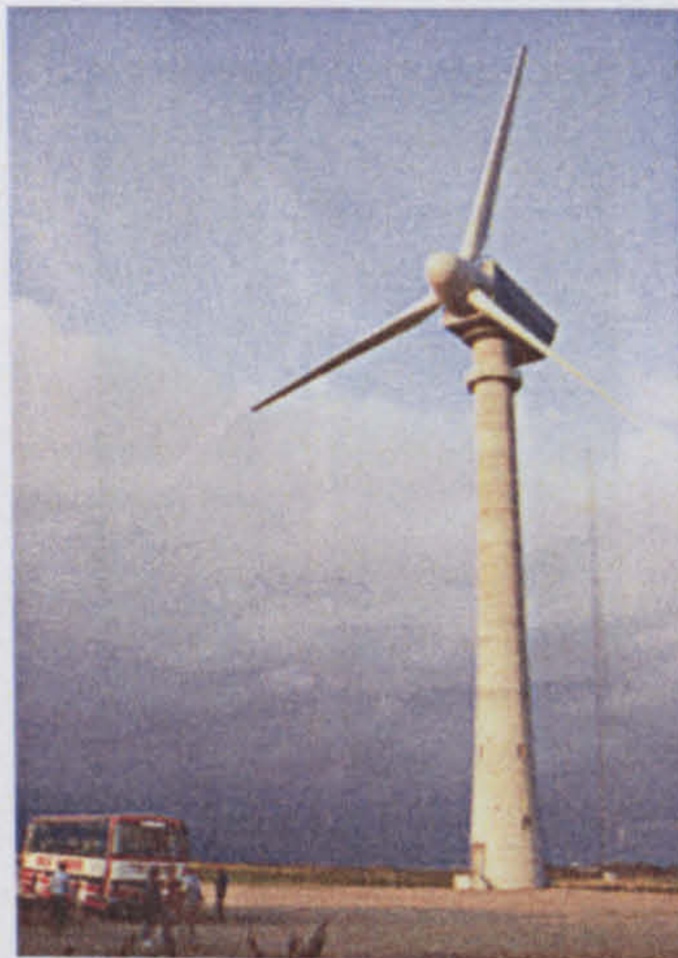
Figure 1.7: A development of the Danish concept WEGA 1; the Tjaereborg rated at 2MW, 1985 [70]
