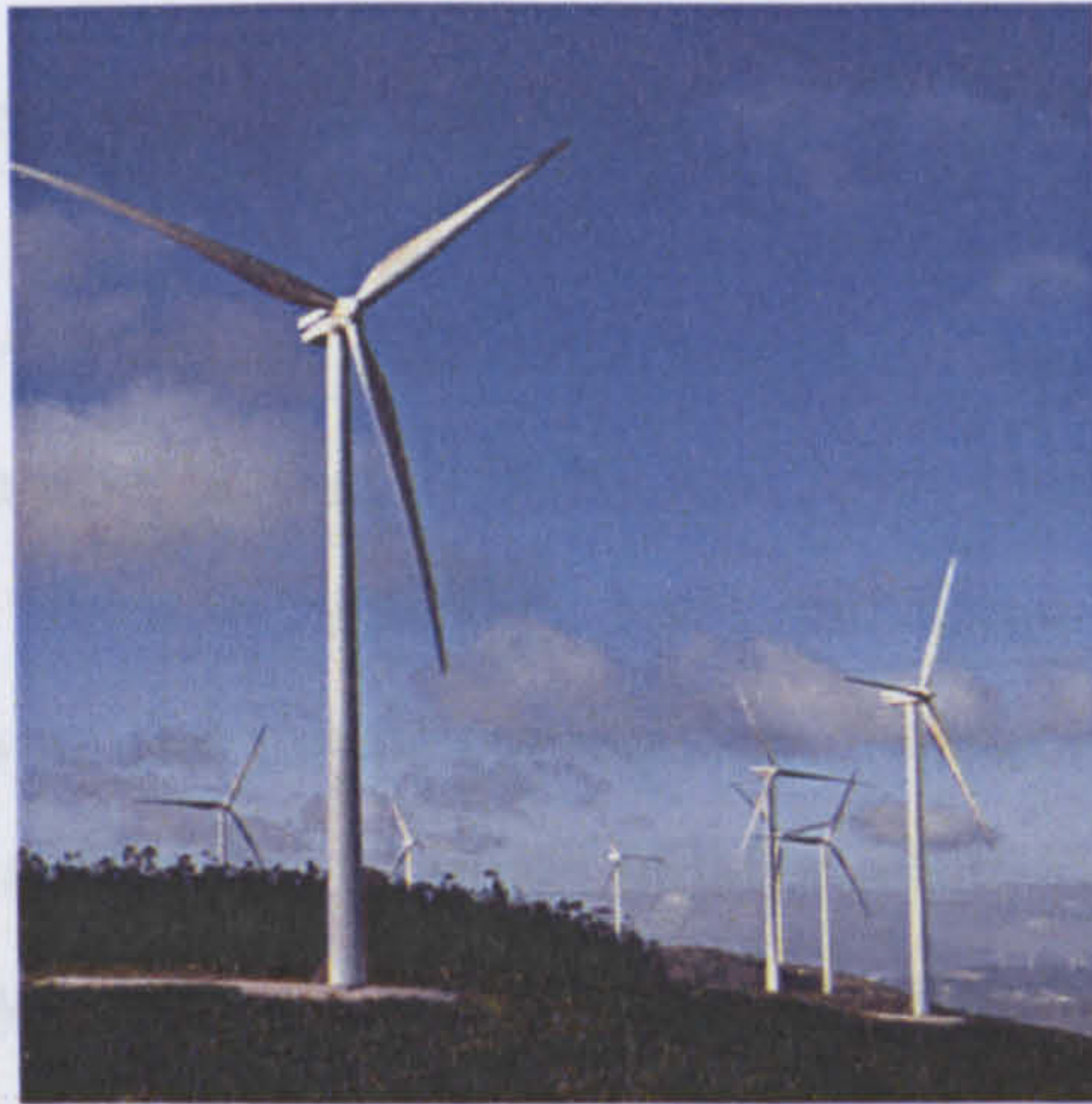
Figure 1.8: A modern Indirect Drive WT, Vestas V90, rated at 3 MW, 2007 [68]
