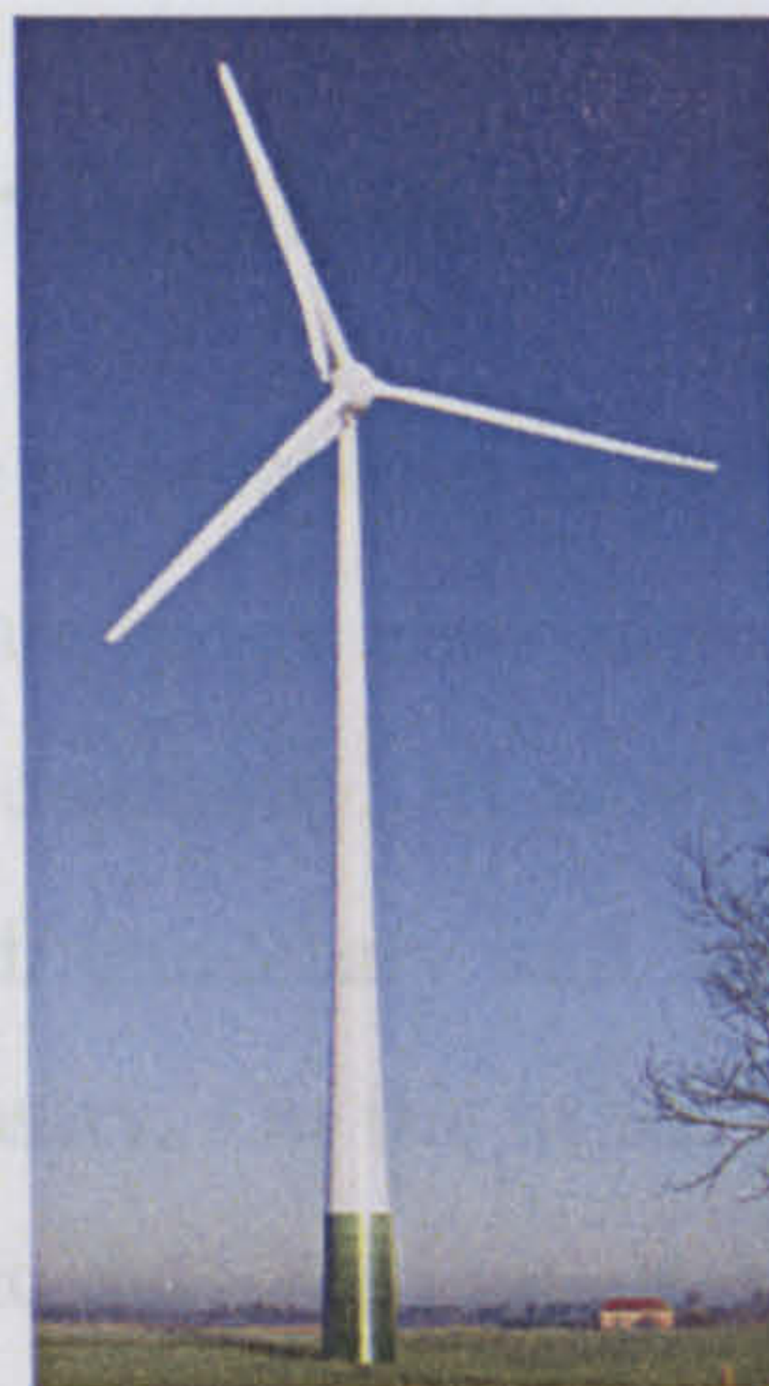
Figure 1.9: A modern Direct Drive WT, Enercon E82, rated at 2 MW, 2007 [69]
