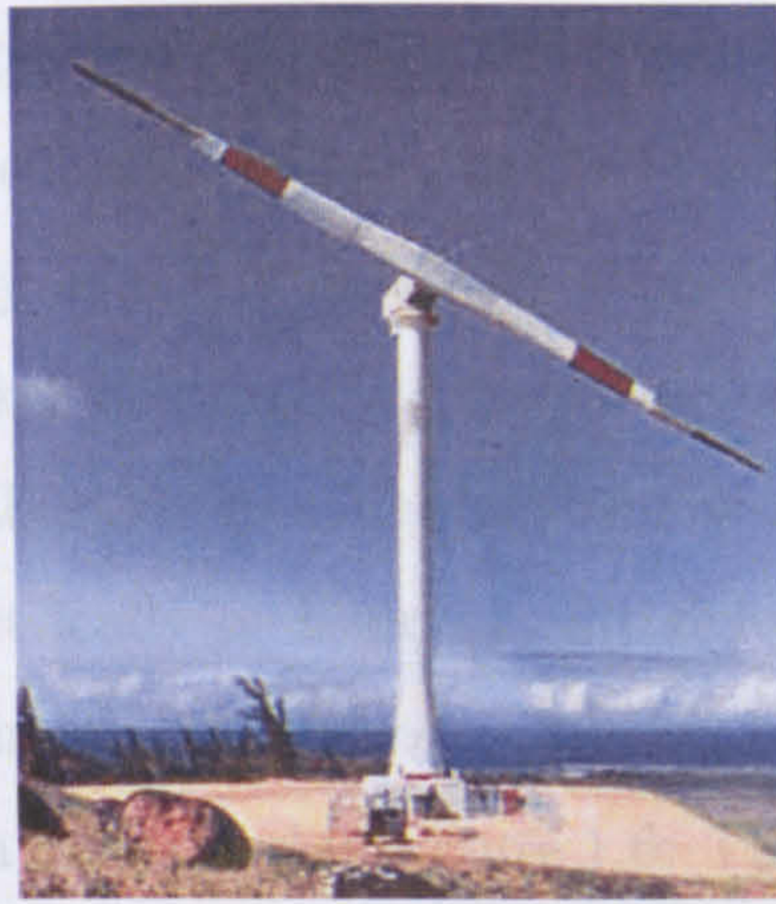
Figure 1.5: The MOD-5, the last product of the U.S. FWEP, rated at 3.2 MW, 1987 [24]
