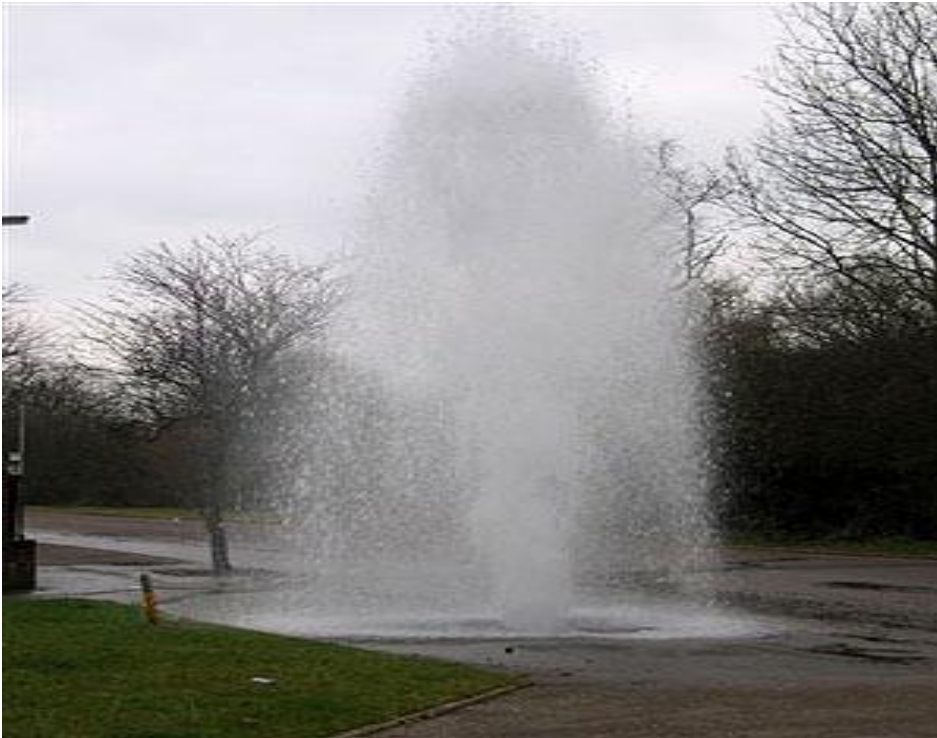
Figure 3-8 Burst in pipe caused due to undetected leak (BBC London, 2009)
