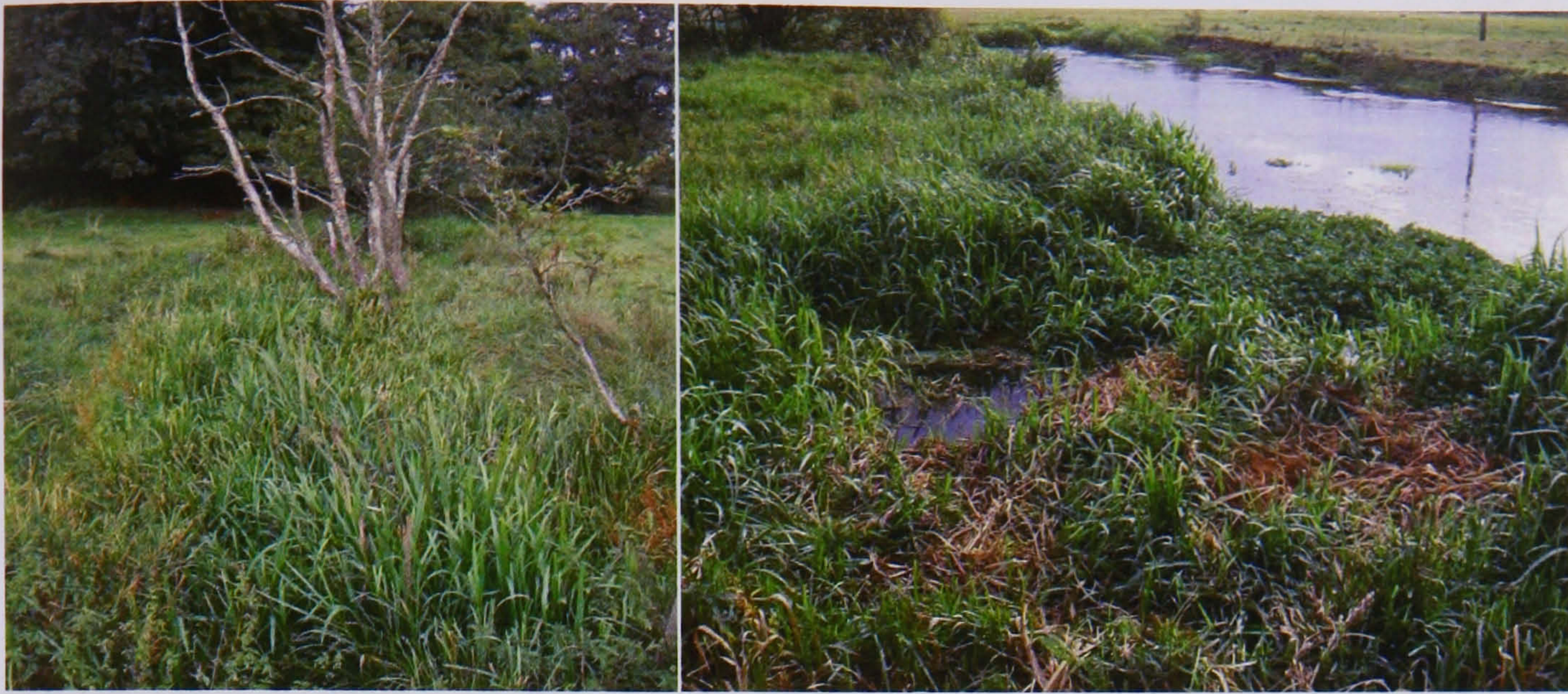
Figure 2.14 Flood relief channel prior to reopening and clearance. Left panel shows the dense emergent vegetation in the flood relief channel and right panel shows the blocked connection with the main river.
