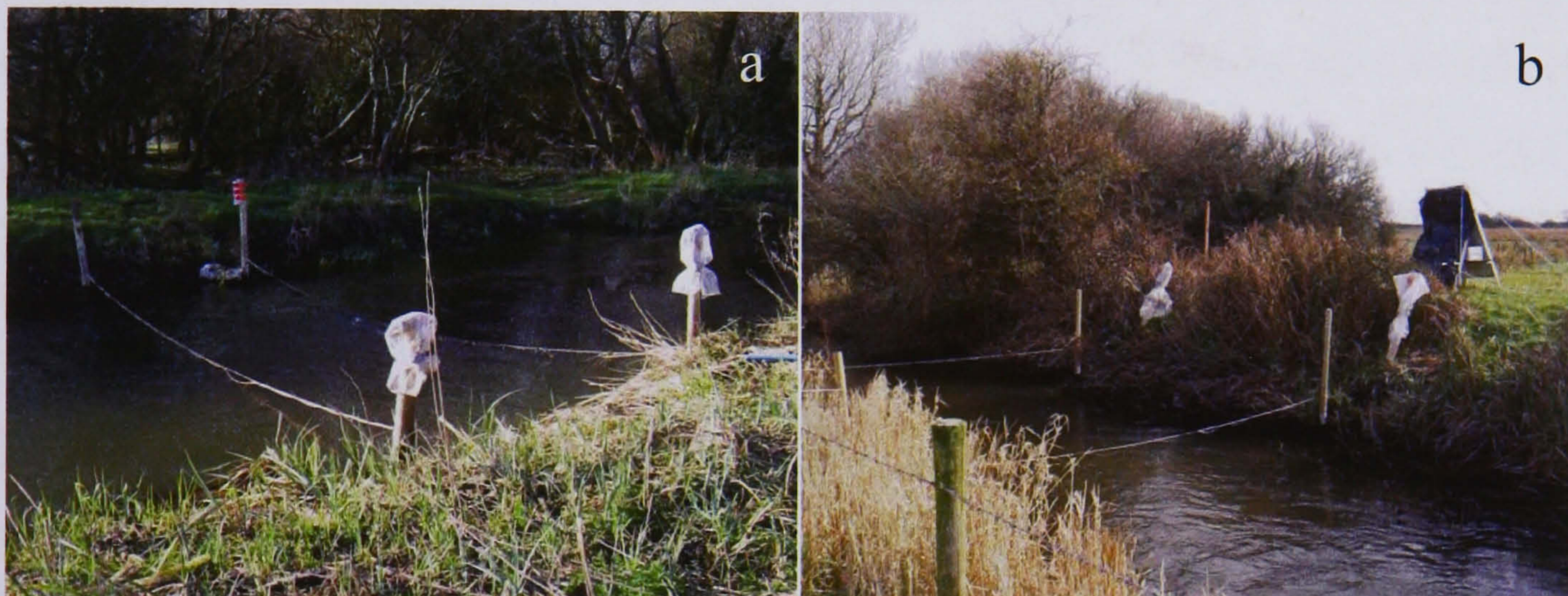
Figure 3.8 TIRIS PIT detectors at the (a) Millhead and (b) Millstream. The solar panel supplementing the two 110Ah 12V batteries can be seen by the Millstream detector. The bank of tuning capacitors in protective bags can be seen in both.
