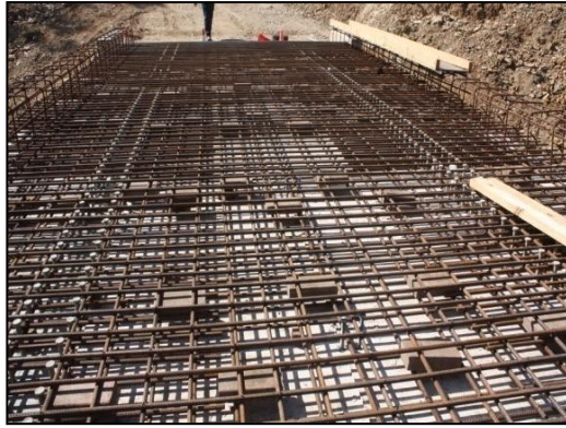
(a) Placing of reinforcement
