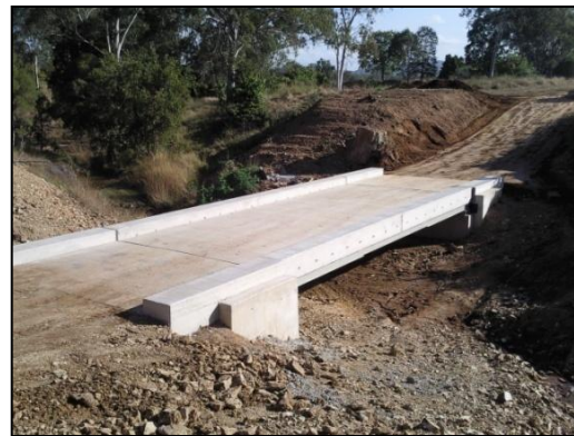
(f) Finished FRW Bridge with RCS deck
