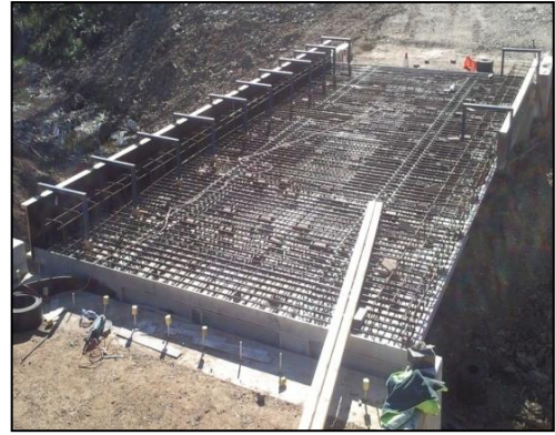
(b) Erection of site formwork for kerb
