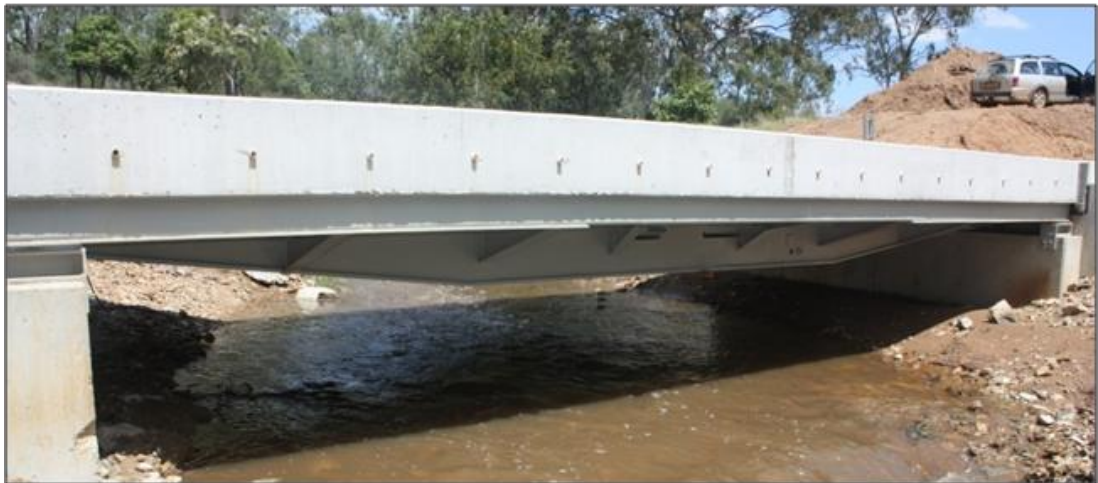
Figure 5.19 Completed FRW Bridge before field load testing
