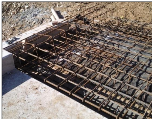
(e) Approach road reinforcement
