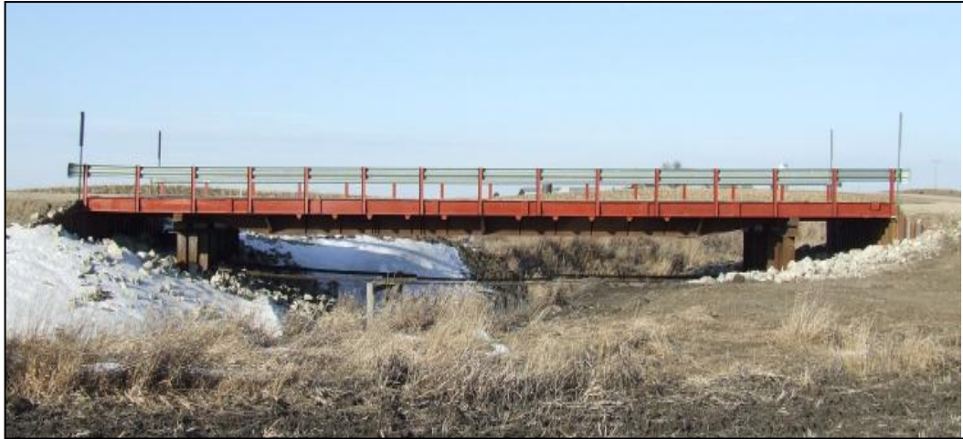
Figure 2.7 Demonstration bridge in Winnebago County (Massa, 2008)
