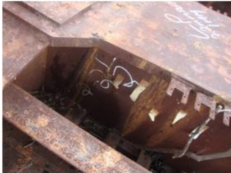
Typical welds on girder top plate
