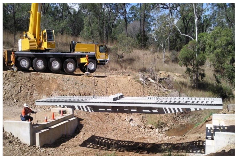
Figure 5.17 Installation of FRWs on the abutment
