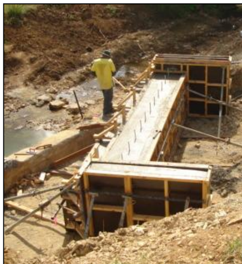
(c) Formwork for abutment
