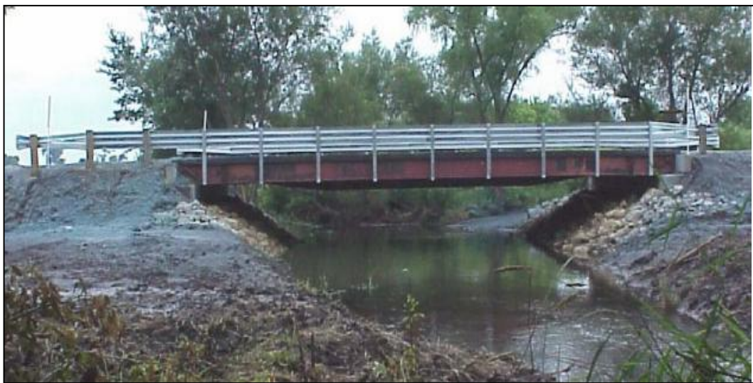
Figure 2.6 Demonstration bridge in Buchanan County (Klaiber et al. 2003)
