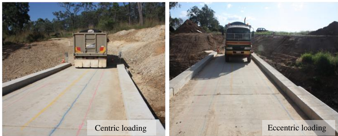
(c) Back view of truck during crawl test
