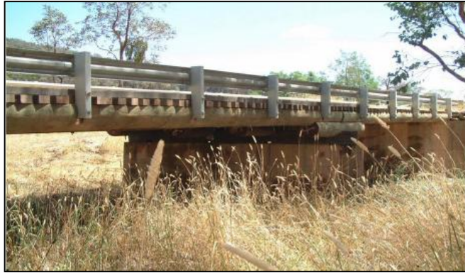
Figure 2.1 Timber bridge on low volume road (Champion et al. 2002)
