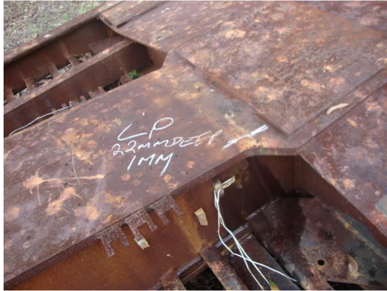
Typical weld 1 & 4 side of centre girder
