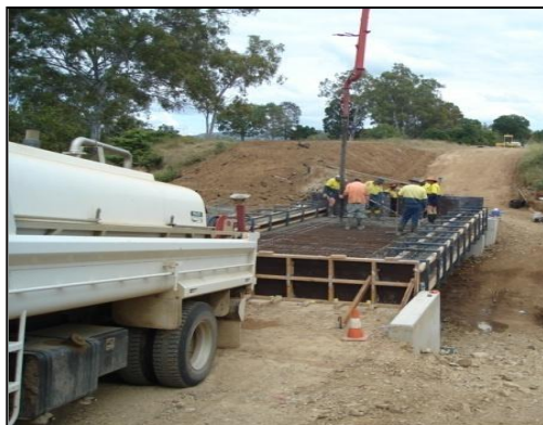
(c) Pouring of concrete from one end
