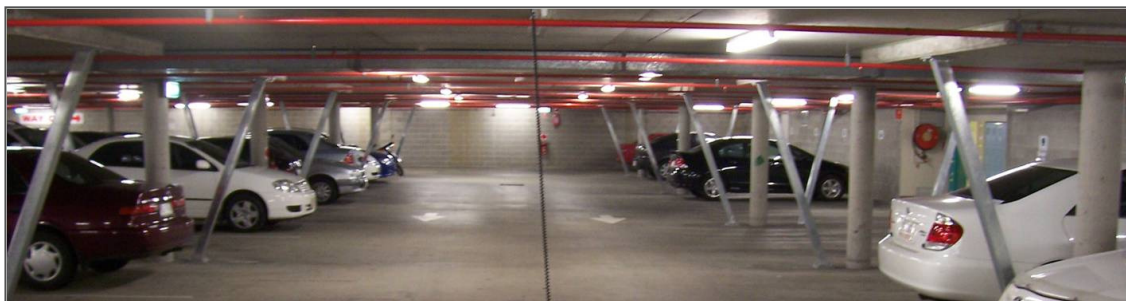
Figure 1.1: Retrofit - structural steel struts installed to reduce vibration
