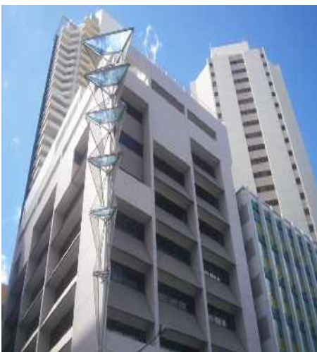
Figure 1 (left) and Figure 2 (right): Office buildings in Brisbane (a sub-tropical climate) employ significant shading strategies to reduce potential glare and solar heat gain, consequently interiors appear dark and gloomy and rely solely on electric lighting.
