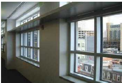
Figure 8: An installed internal light shelf [16]
