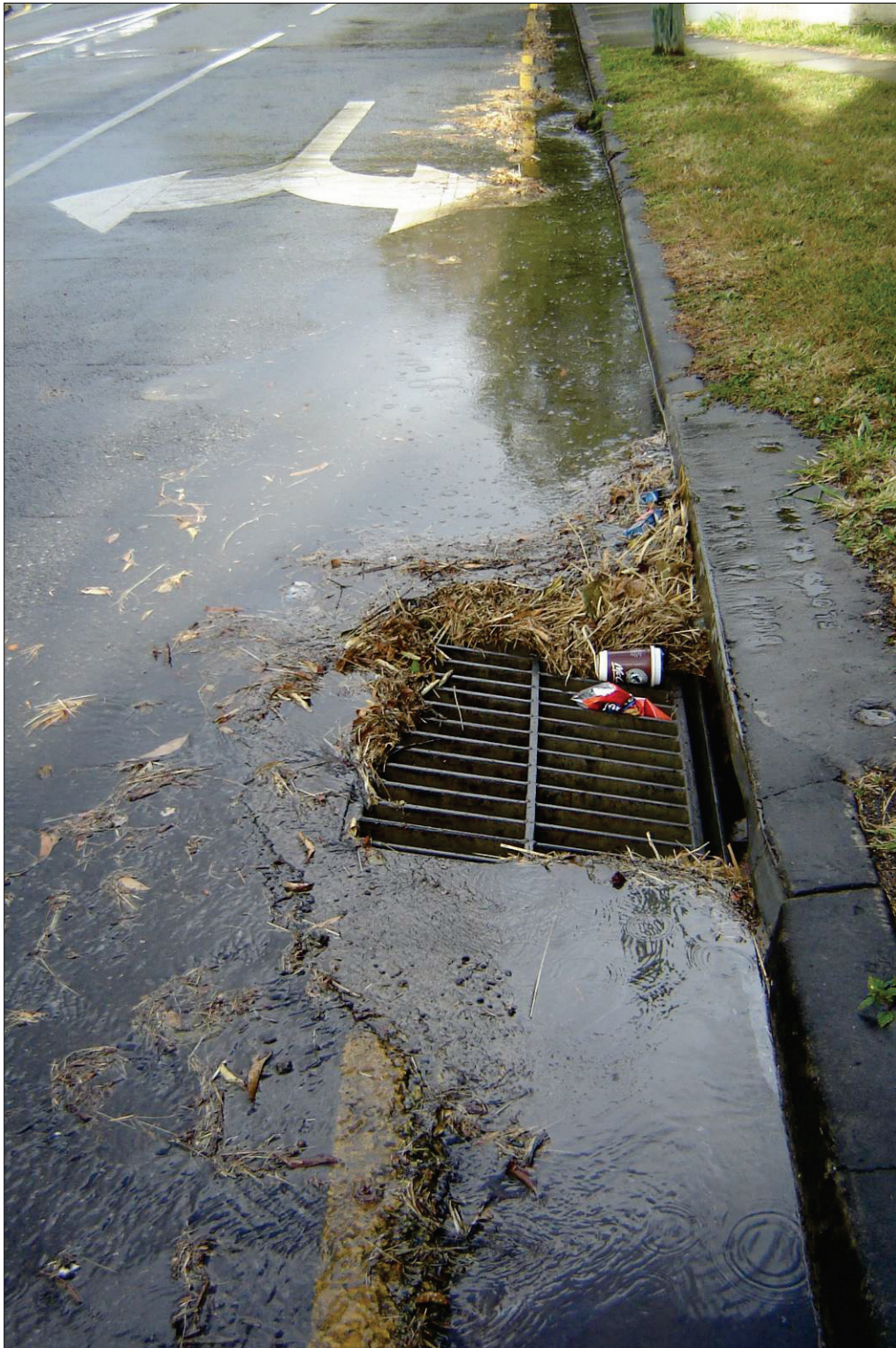
Figure 4.27 An accumulation of organic matter (mainly grass clippings) obstructing the water flow course at the stormwater drain.
