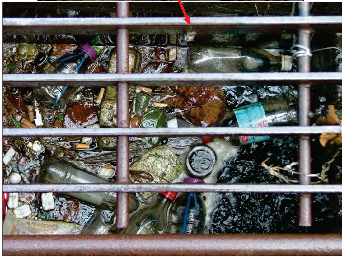
Figure 4.13 A collection of litter (plastic bottles, cigarette butts polystyrene and organic matter) in a stormwater drain (SWD No. 10, See Tables 4.1 and 4.2) during wet weather.
