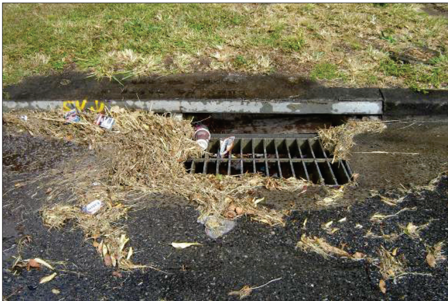
Figure 8.2 Clippings from grass verge collected at a stormwater drain at Park Road, South Brisbane (2008).
