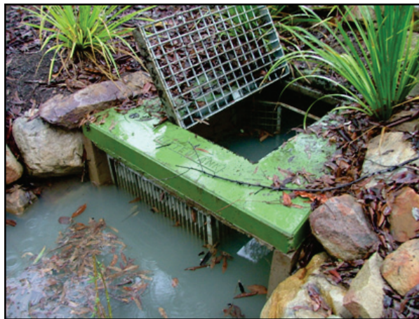
(b) Right, front view of a partially blocked screen with organic matter from incoming stormwater.
