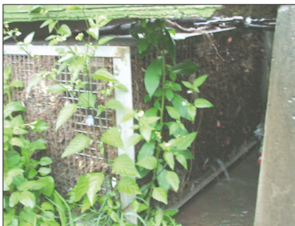
Figure 8.4 Field surveys showing the GPT LitterBank with (a) high, and (b) low water tidal levels, partially and (c) fully blocked screens.
