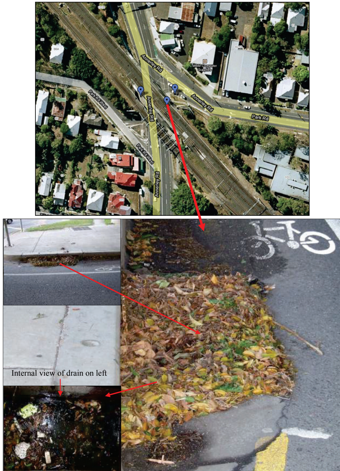
Figure 4.11 A storm water inlet drain (SWD No. 19, See Tables 4.1 and 4.2) on a busy route under a railway bridge is covered with organic waste (at the T junction between Park Road and Annerley Road, South Brisbane). Lower left is inside the drain which is blocked with stagnant water contaminated with traffic dust. The upper left is the front view of the drain located at the junction (May 2008).
