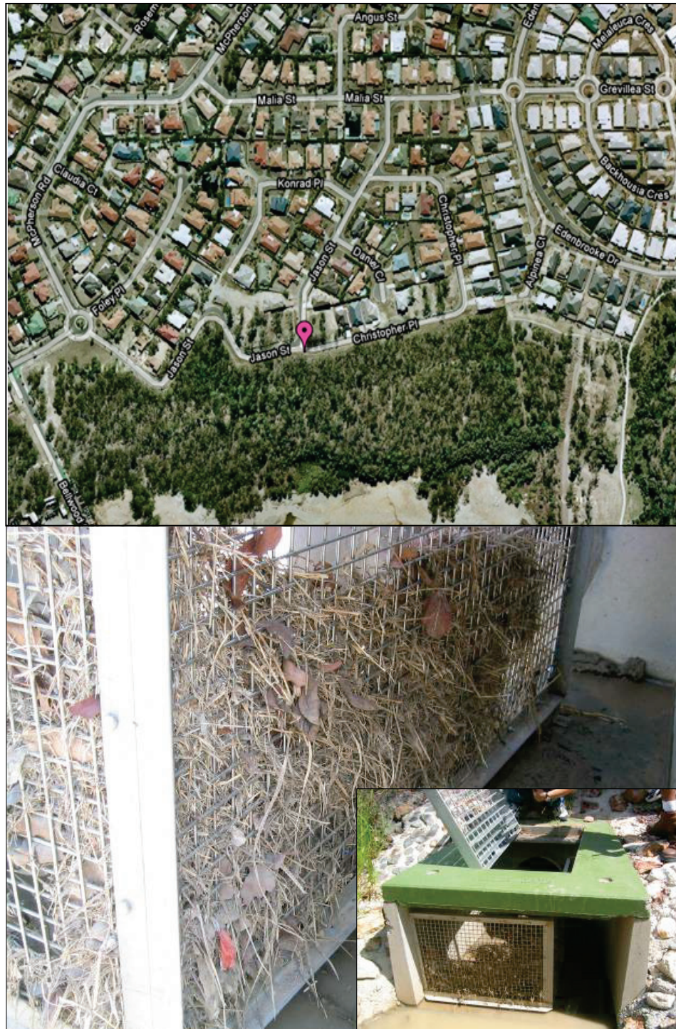
Figure 4.22 Lower right is a gross pollutant trap for the nearby housing estate (Sinnamon Park an outer suburb of Brisbane) catchment. Gross pollutants captured mainly consist of organic matter such as leaves and grass clippings which clog the internal retaining screens.
