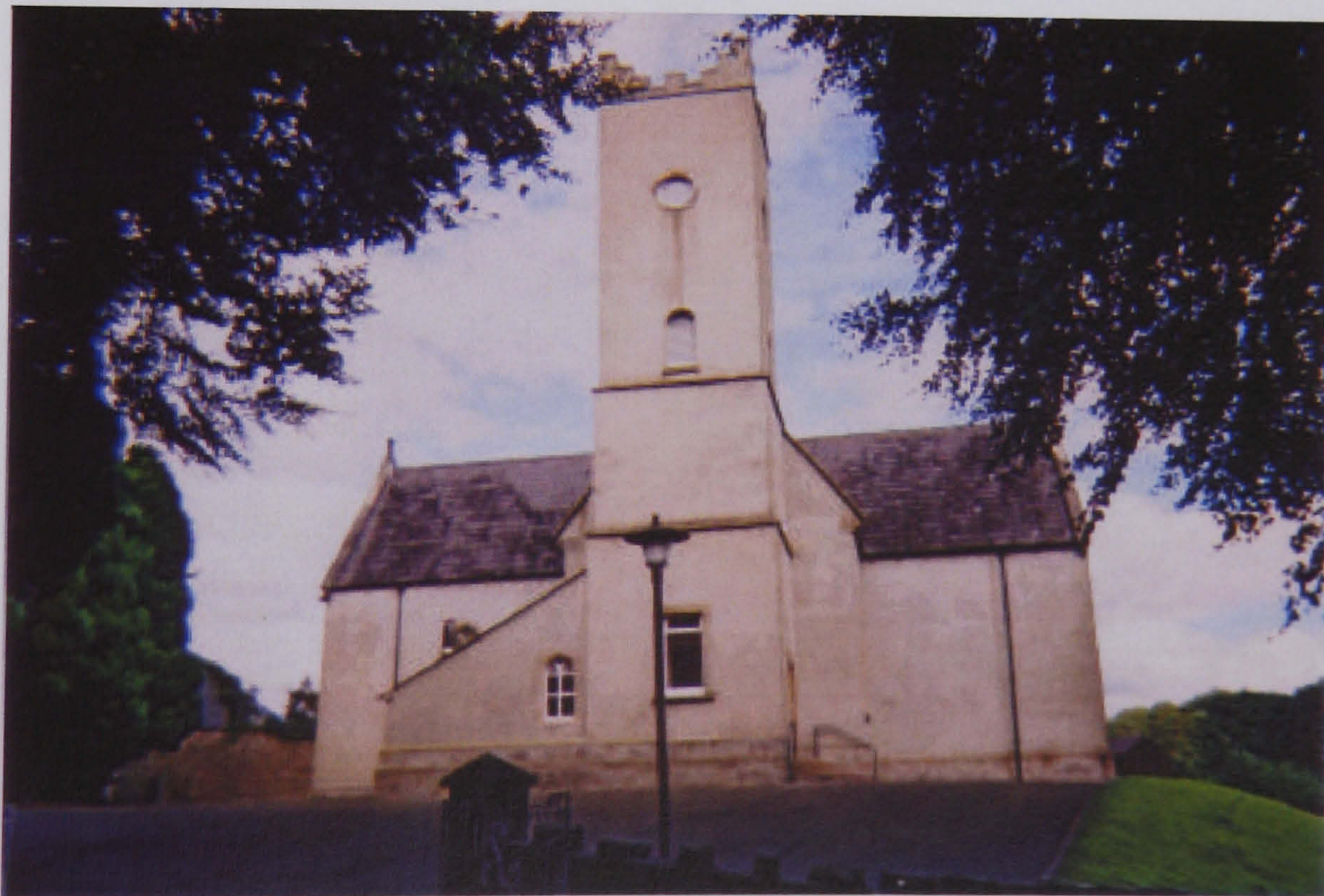
Plate 11:2 Drumkeeran Parish Church, Tubrid, County Fermanagh
