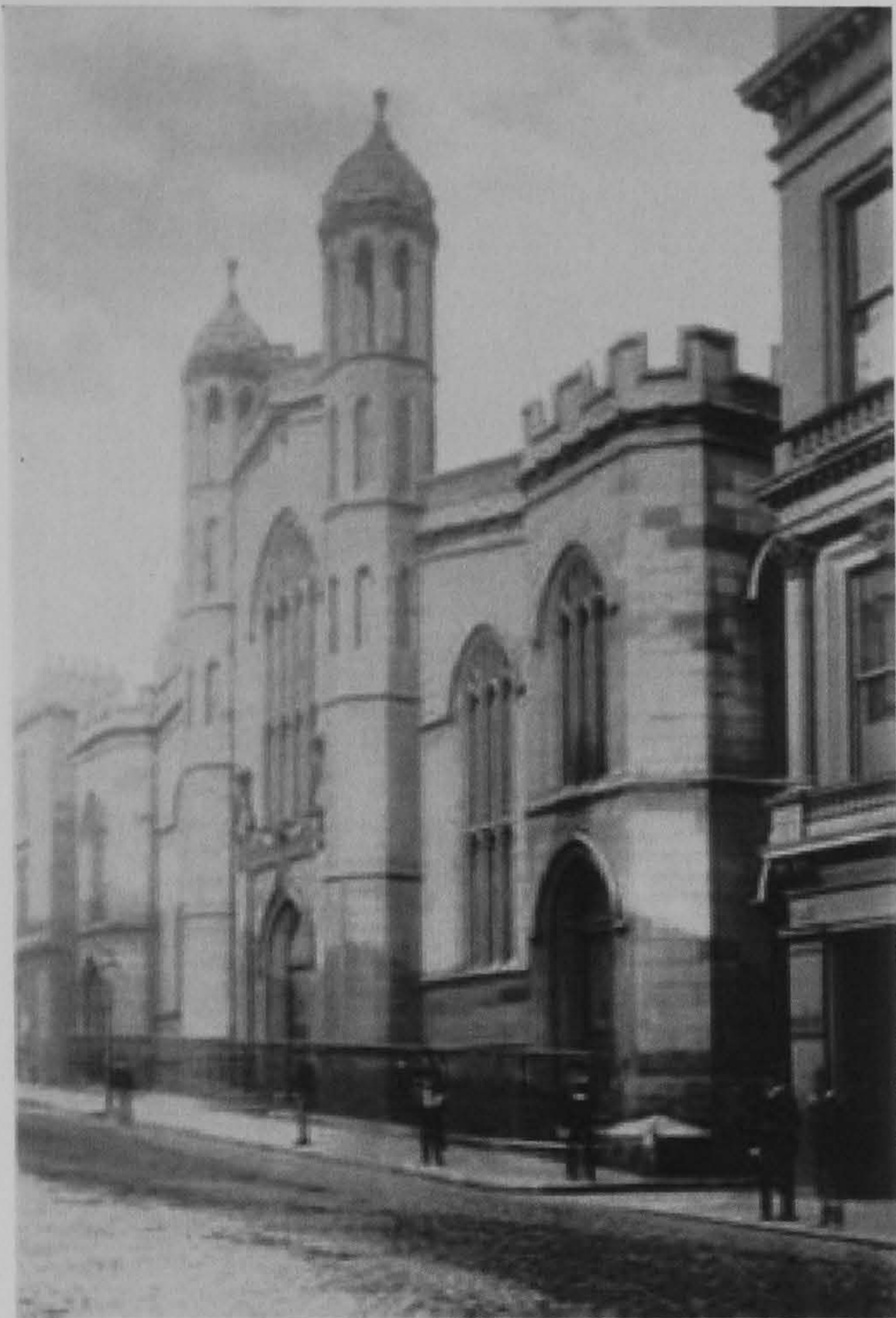
Plate 6:1 St. Mary's Renfield St, Glasgow
