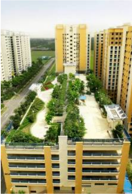
Figure 4: An intensive green roof added to an existing carpark, Punggol housing estate, Singapore (Photo: National Parks Board, Singapore)
