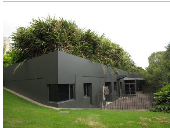
Figure 6: Densely planted intensive green roof on Sydney Conservatorium of Music (Source: the author, 2008)
