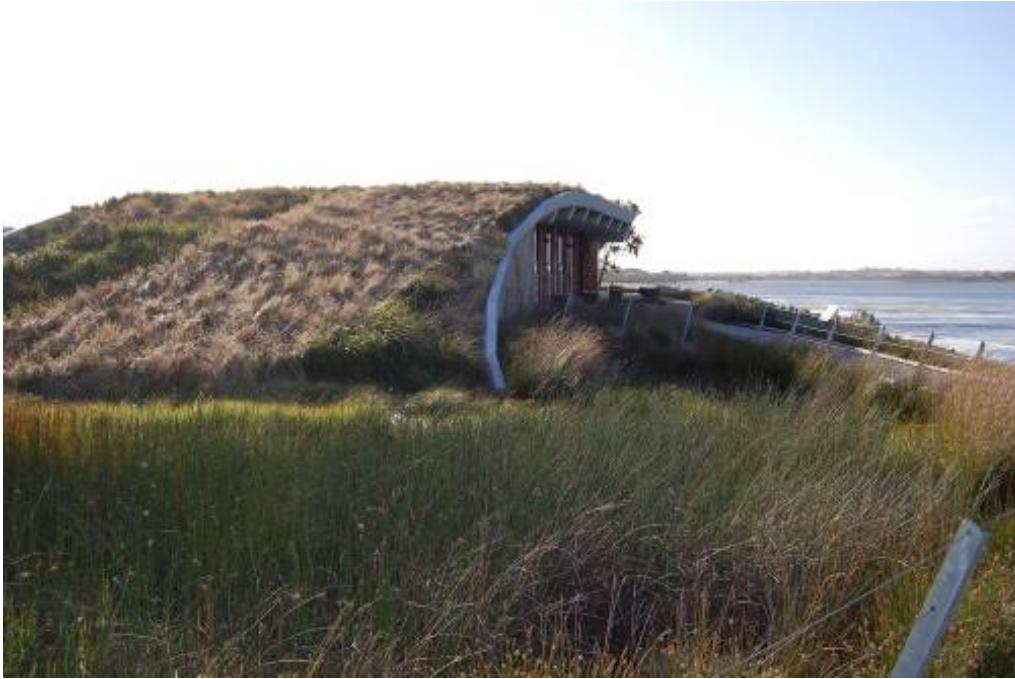
Figure 3: Marine and Freshwater Resource Institute of the Department of Public Infrastructure in Queenscliff, Victoria (Photo: Sidonie Carpenter, 2008)
