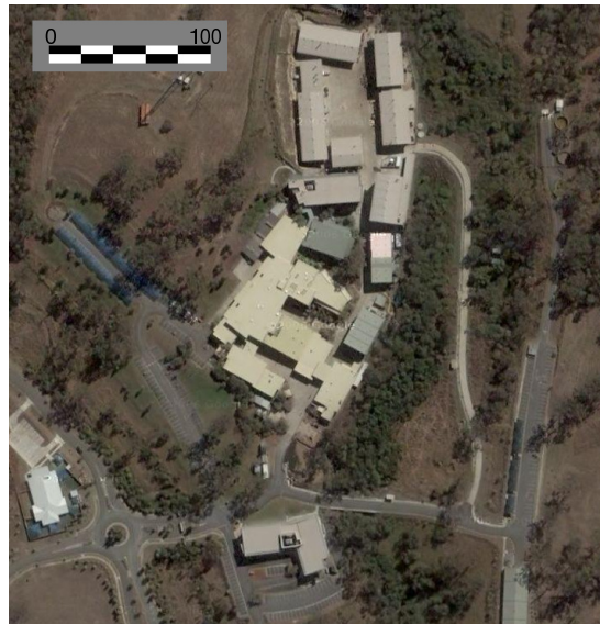
(a) Aerial view of Queensland Centre for Advanced Technologies (QCAT). The scale in the upper right corner is distance in metres.
