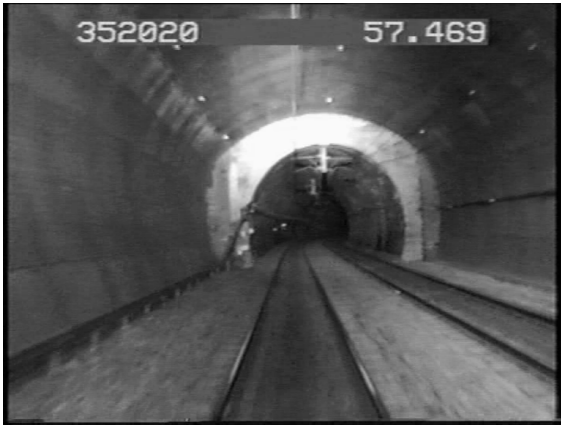
Fig. 2. An image from a tunnel. The rails are dark.
