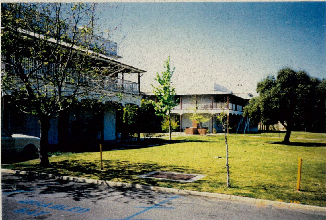
ADMINISTRATION AND RESIDENTIAL PROPERTIES OUTSIDE WALLED SECTION
