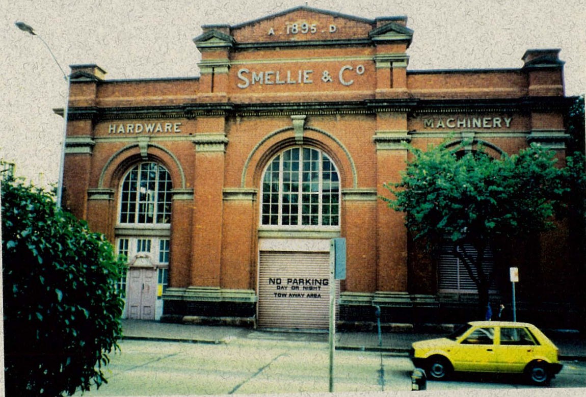
SMELLIES' 'RED BRICK' BUILDING - EDWARD STREET
