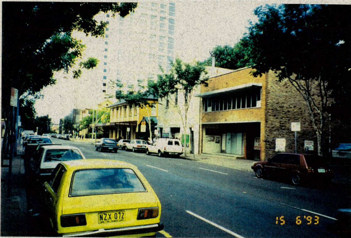
MARGARET STREET STREETScape - SHOWING, LEFT TO RIGHT, PORT OFFICE HOTEL, OLD ST VINCENT DE PAUL HOSTEL, WORKSHOP BUILDING AND LAND
