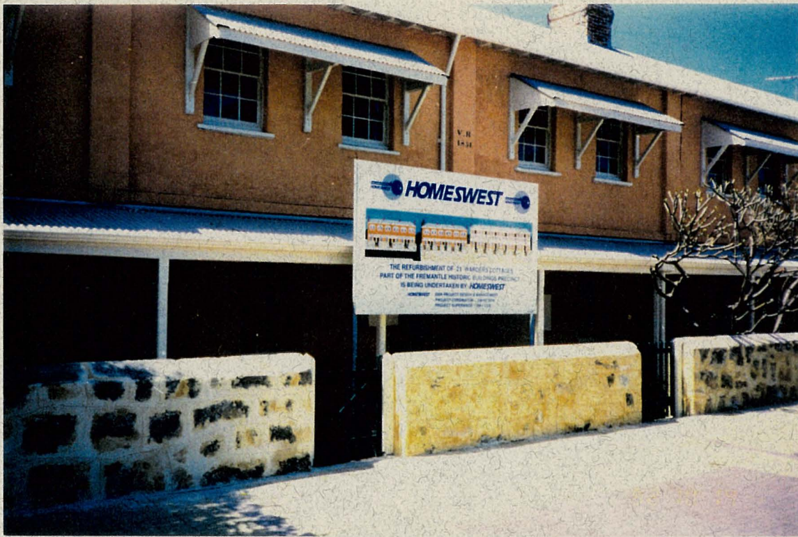
RESTORED WARDER'S COTTAGE - OFF SITE
