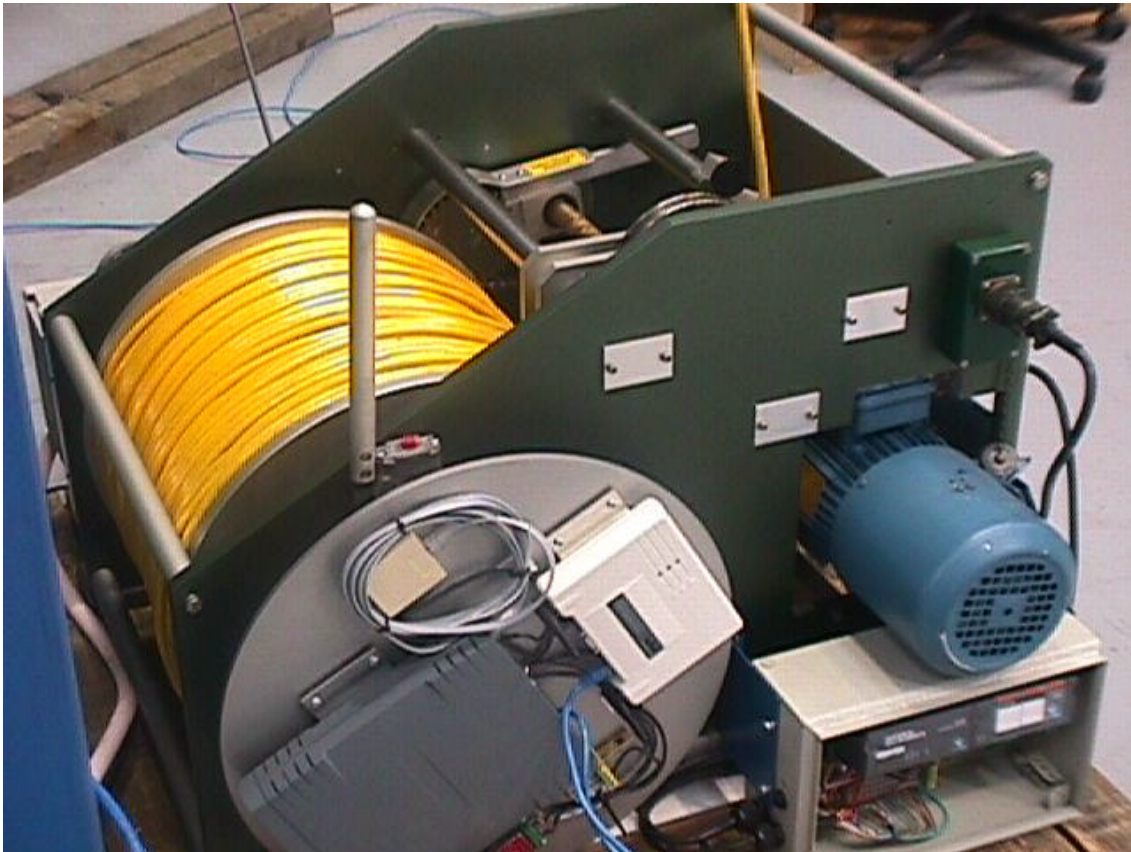
Fig. 1. CISCO 802.11b access point connected to a HDSL modem mounted on a rotating cable reel.
