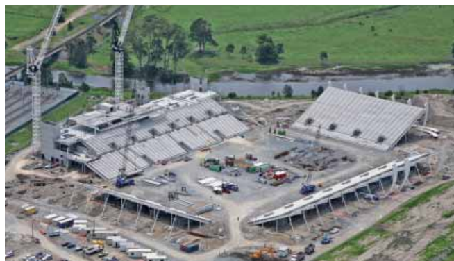
Robina Stadium site January 2007 (Source: Watpac Construction)
