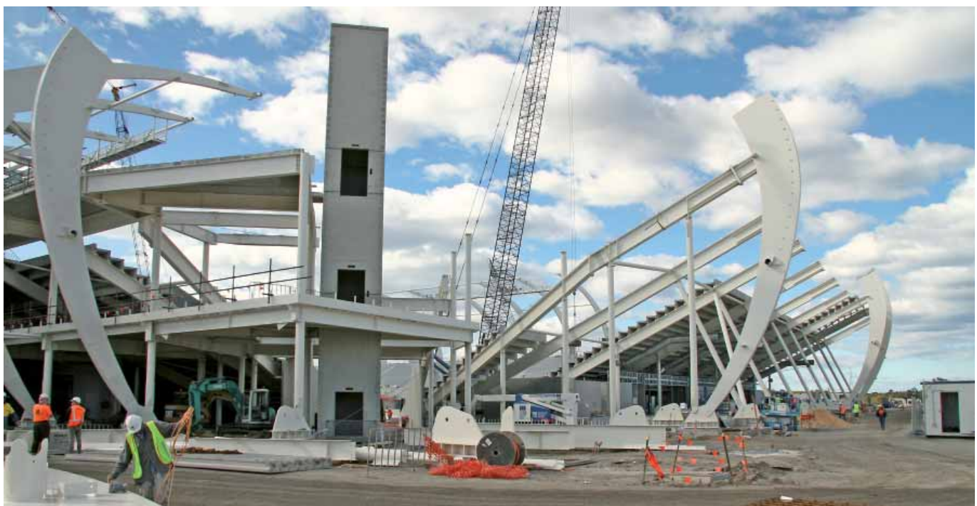
Off-site manufactured steel structures in place
