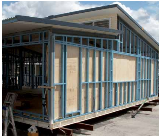
With completed roof in place the framework and fitting out commences
