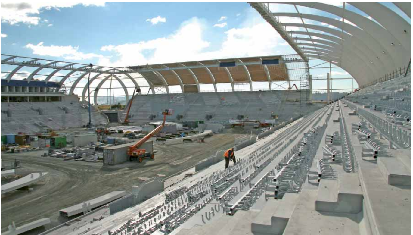
Concrete plats receiving seating
