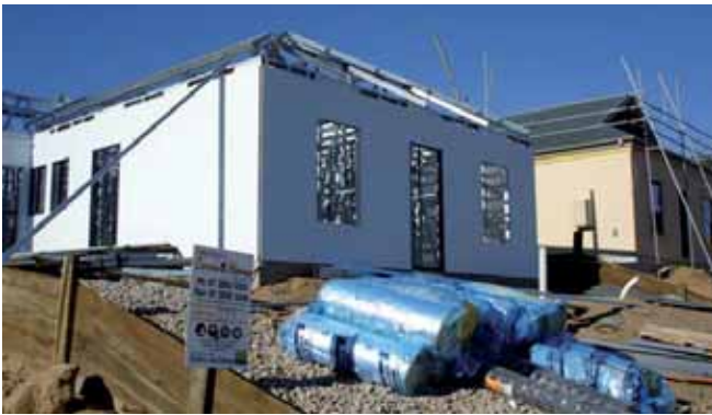
Construction on site (Source: Monarch)
