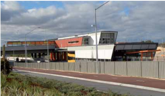
Near complete station with footbridge to the left (Source: New Metrorail 2006)
