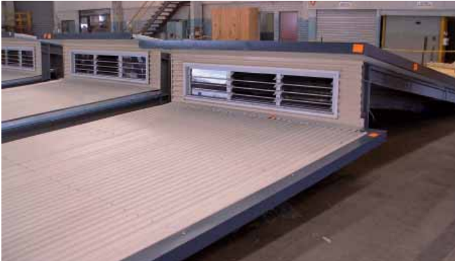
Completed roof sections assembled at ground level
