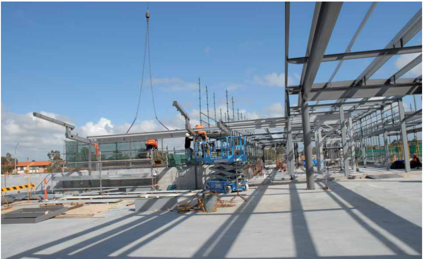
Prefabricated steel section being placed (Source: New Metrorail 2006)
