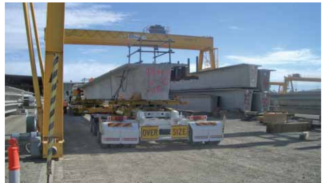
Jinkers being loaded with post-tensioned bridge beams
