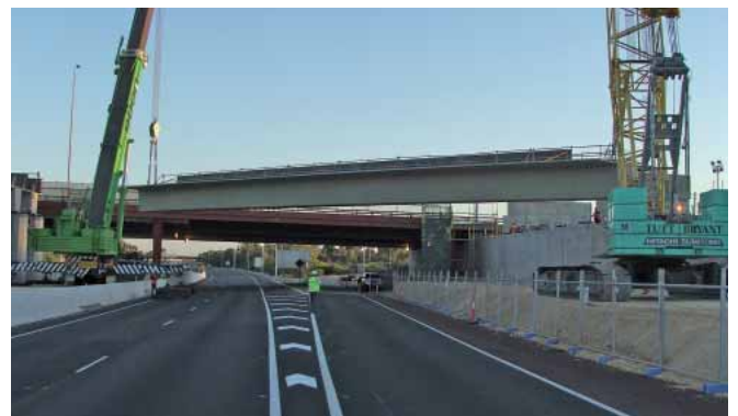
Leach Highway bridge T-Roffs being lifted into position (Source: New Metrorail 2006)
