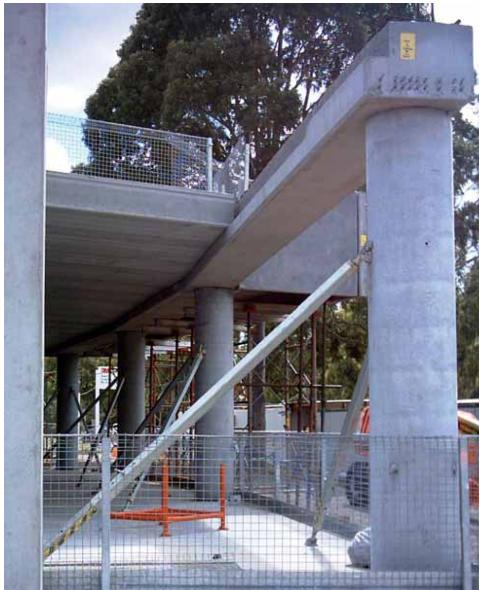
Hollow-core planks, beams and columns (showing support) on site (Refer page 31)
