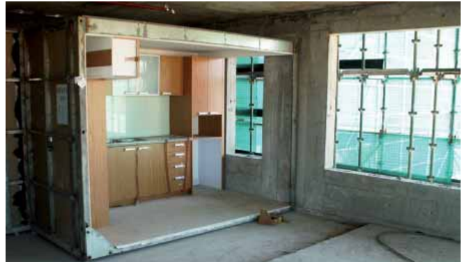
Kitchen module in place by window (note drop down floor)
