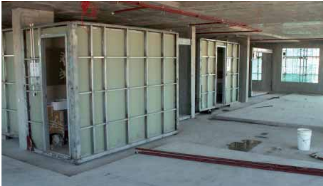
Modules in position (note void above for services)
