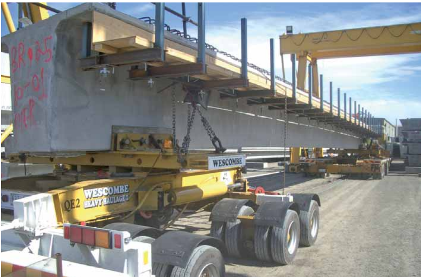
Safety rails fitted to beam and loaded onto jinker for transportation
