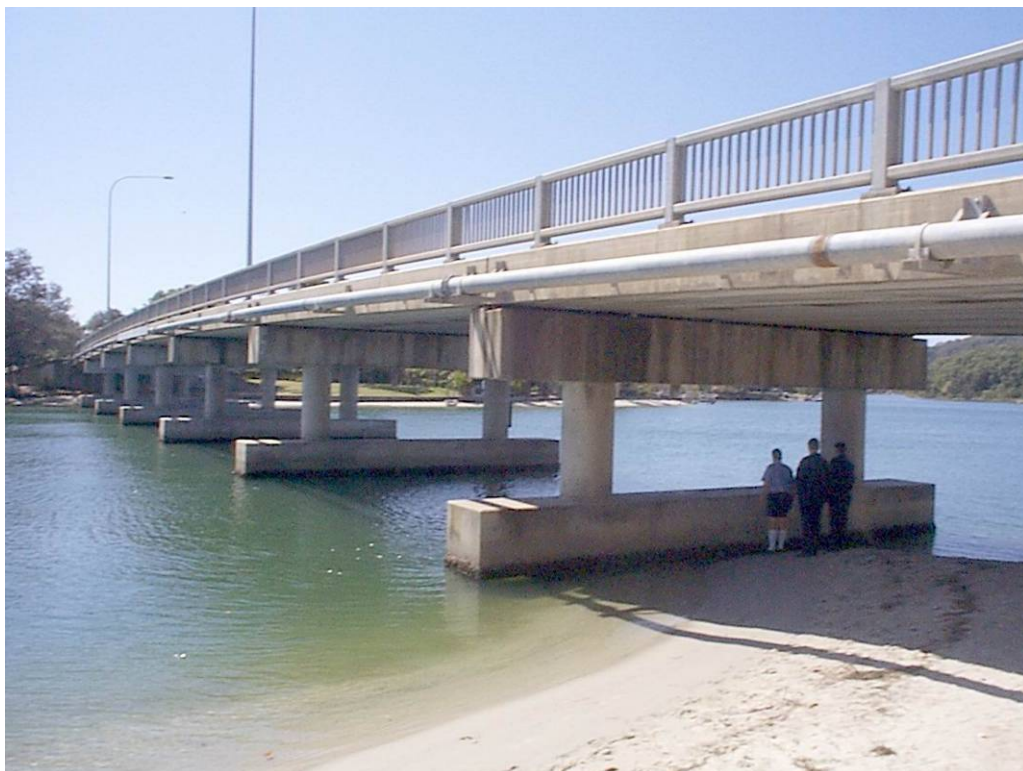
Photo 1. General view of Bridge 1
