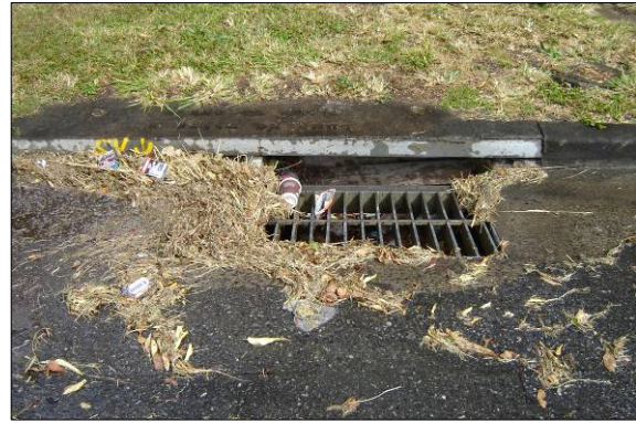
Fig. 2: Clippings from grass verge collected at a stormwater drain at Park Road, South Brisbane (2008)
