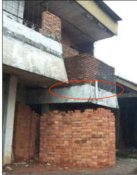
Figure 2.11 Masonry wall and brick deposit (Bandung)
