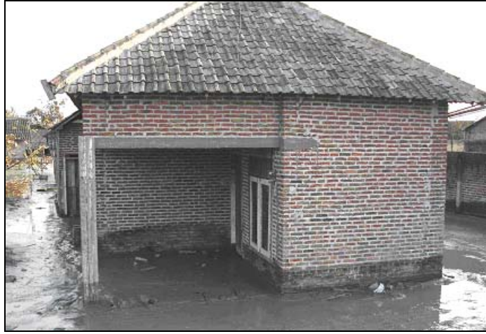
Figure 2.13 Masonry house without tie beam and column, viewed from front (Porong – 2006)
