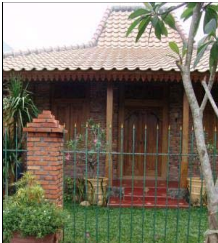
Figure 2.2 Brick house in Bali
