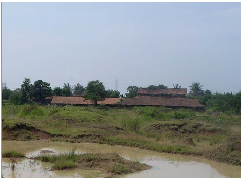
Figure 2.16 Clay brick factory in Cikarang – Jakarta
