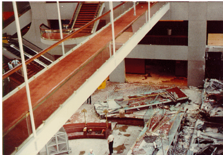
Figure 1-1: After Hyatt Regency Hotel walkway collapse in Kansas City in 1981
