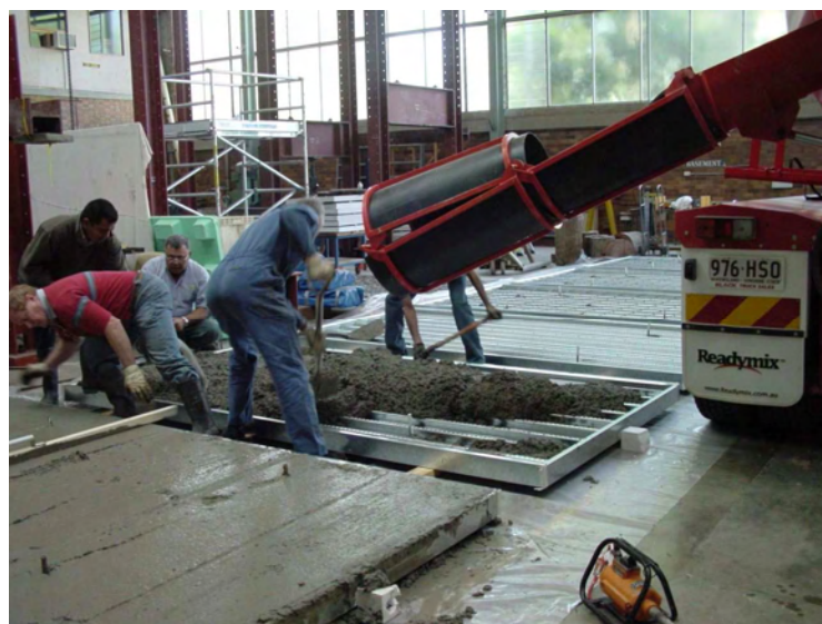
Figure 3-11: Casting, trimming and spreading concrete
