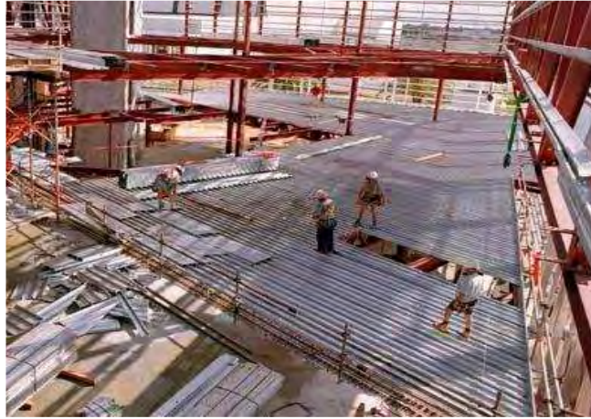
Figure 4-1: Steel-deck floor panels being sep up for construction (BlueScope Lysaght)
