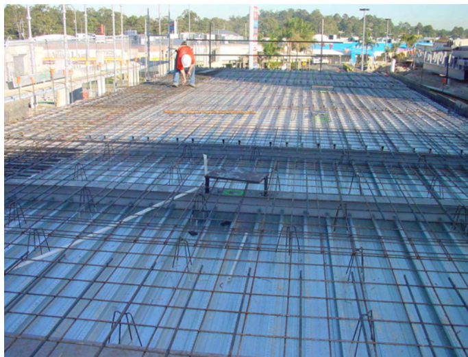
Figure 1-4: Composite floor construction in a shopping mall, Logan City Hyper-dome, Brisbane
