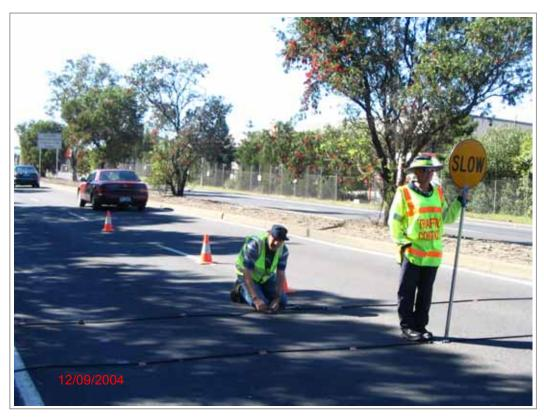
Figure 6.11 – Installing the automatic traffic counters
