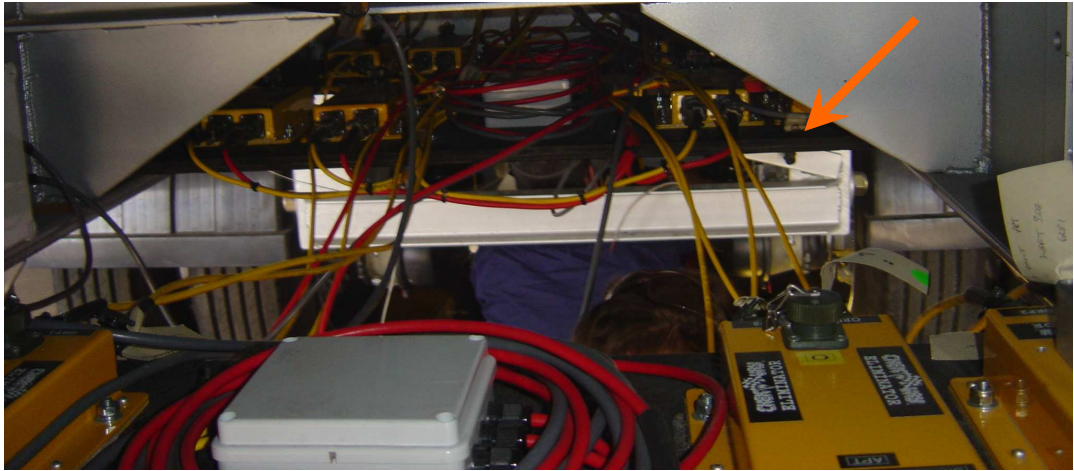
Figure 16. View underneath of semi-trailer, looking to rear.
