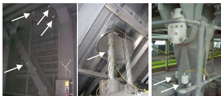
(1) Truss Girder (2) Hanger Cables (3) Rocker Bearing
