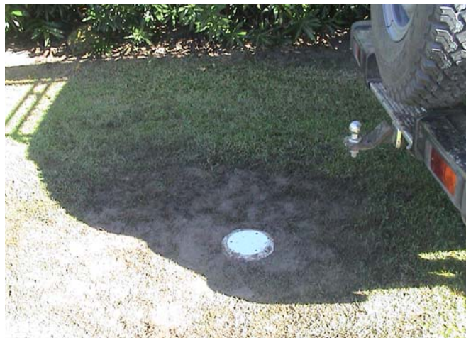
Figure 3.3: Well security achieved by placing sealable concrete caps over monitoring wells flush with surface
