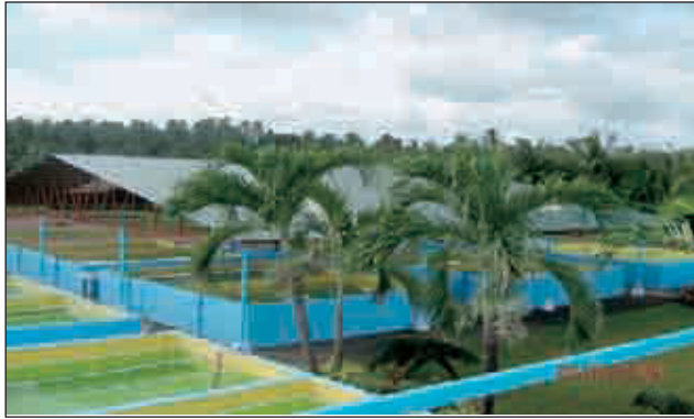
Community grouper cages and marine fish hatchery in Misamis Occidental, both assisted by AQD in design & construction, operations and skills training
