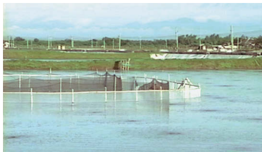
Center Sludge Collector
