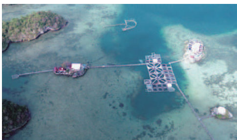
Igang Marine Substation
