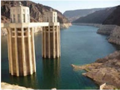
Figure 12: Electrical power station in Hudson river, in Nevada (US). This power station gives all the electrical energy that Las Vegas needs
