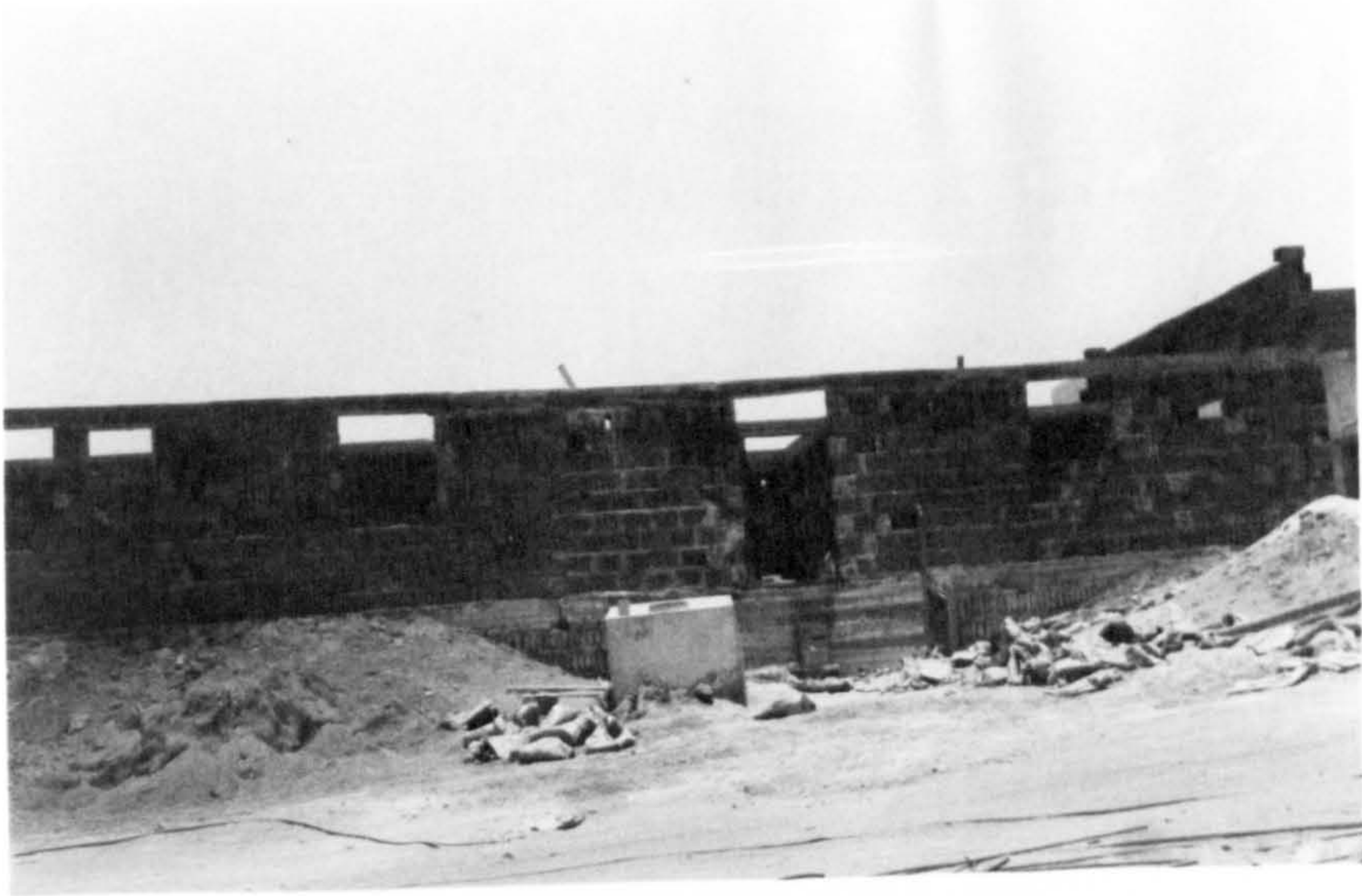
Plate 7.9 : A stage in the construction of a squatter house.
