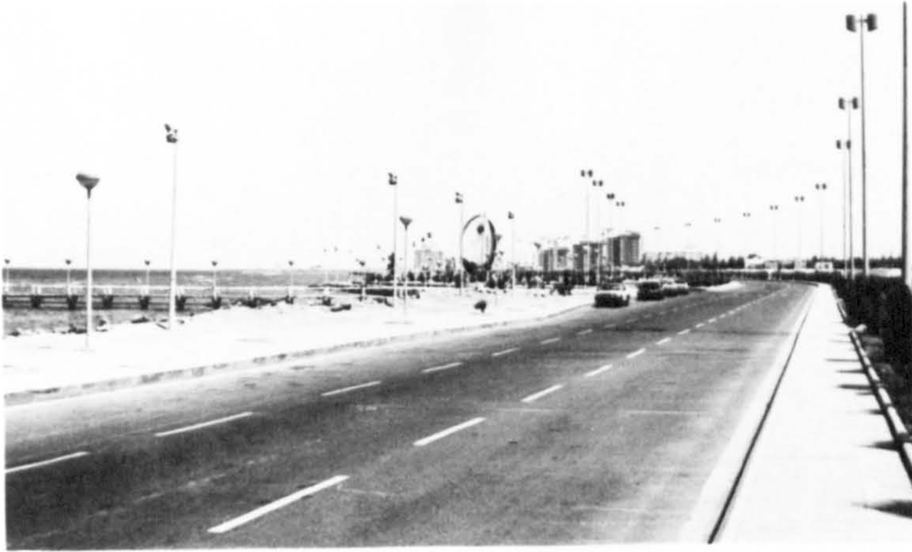
Plate 8.1: Al-Cornich Street: One of the main internal highways.
