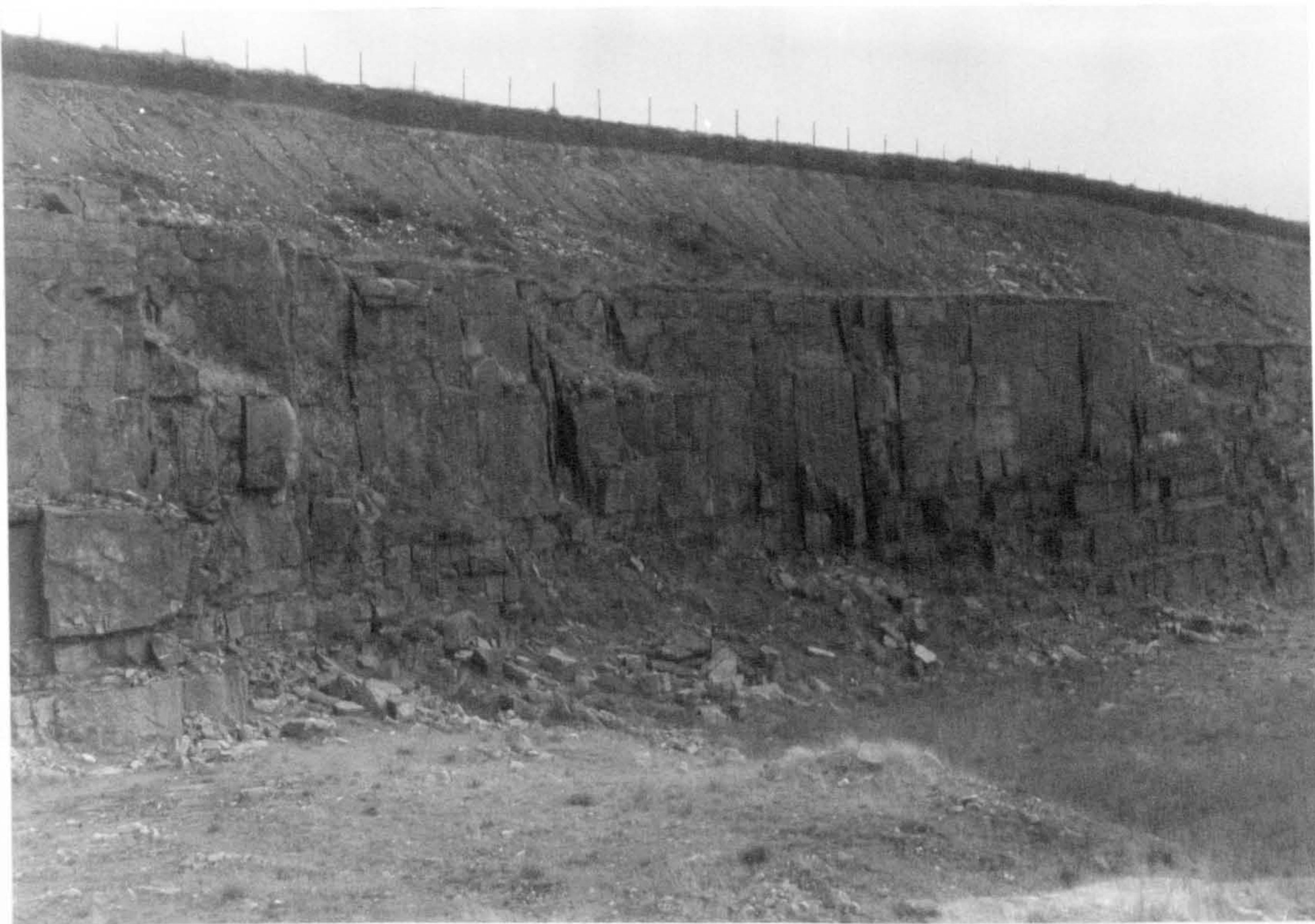
Thickly Bedded Facies exhibiting low angle depositional dips, Harthope Bank Quarry. Quarry face approximately 7m. high and orientated N.W.-S.E. (left to right).
