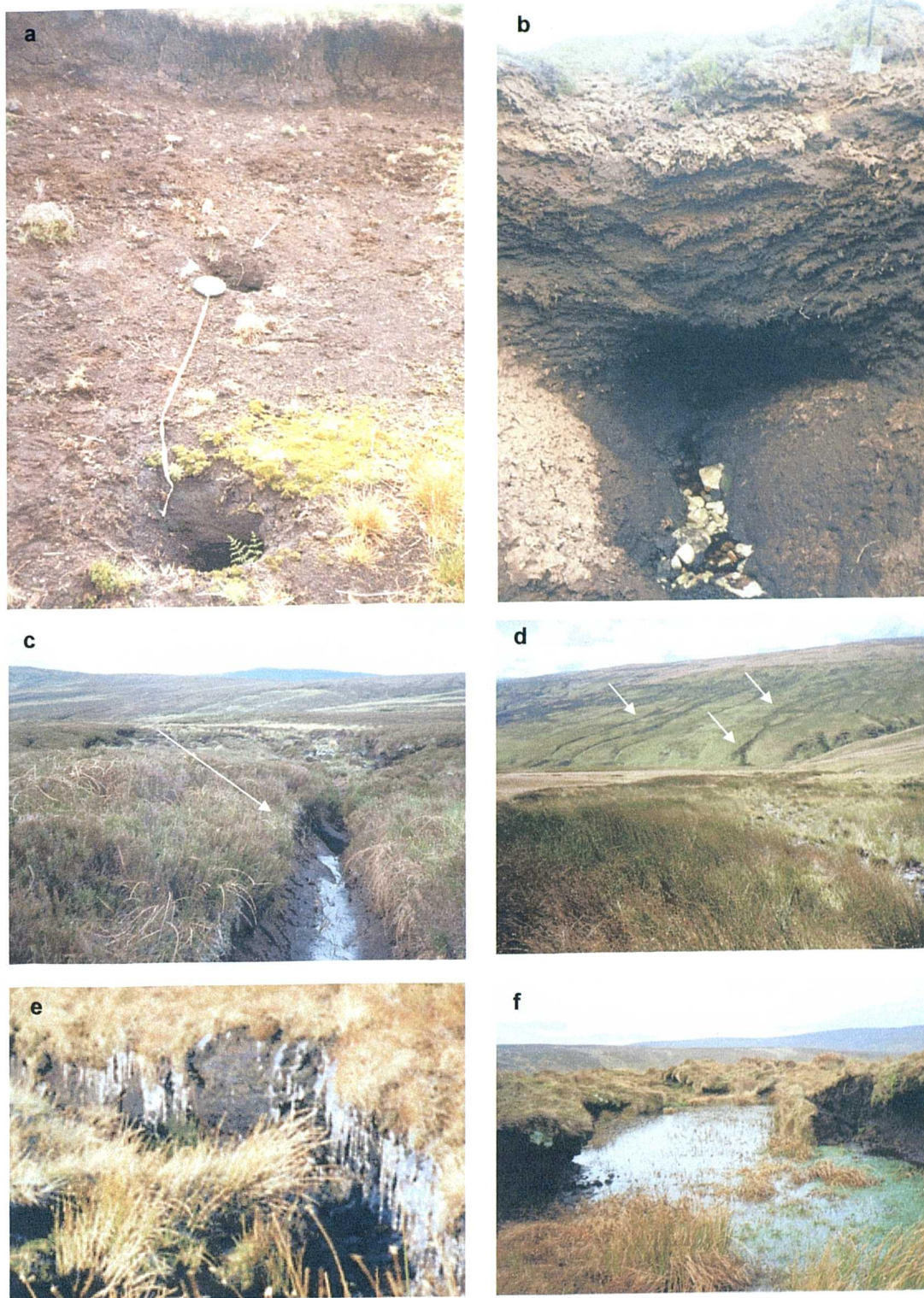
Figure 3.7. Drainage features associated with peat slides and bog bursts. a) karstic pipe network revealed in lower excavated part of Glendun bog burst; b) large pipe, (note spade for scale) in deep peat on Meldon Hill; c) grip feeding the head of Beagh's Head (Co.Antrim) bog burst; d) linear flushes feeding valley side gully network on slope opposite Middlehope peat slide (foreground); e) icicles indicating extent of former acrotelm surface flow at Langdon Head peat slide; f) ponding and vegetation development between raft-jam at Nein Head 2 peat slide.
