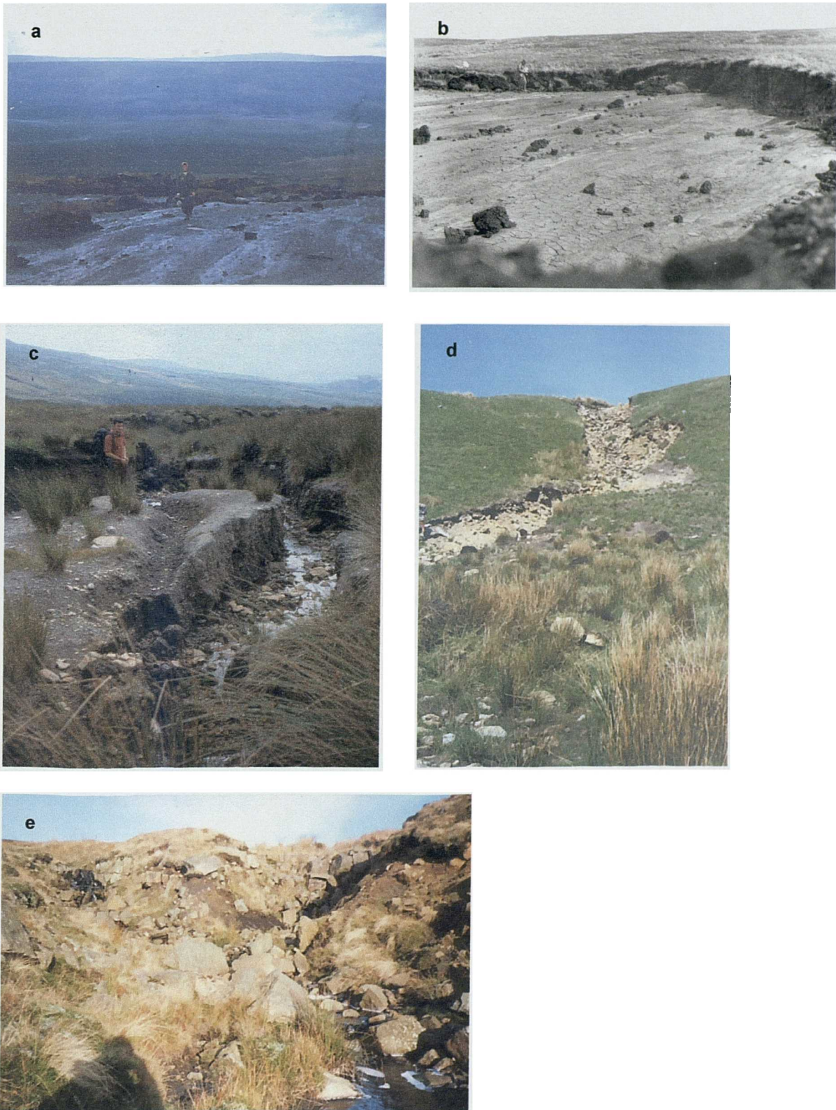
Figure 7.10. Contrasting drainage patterns with increased scar exposure.
