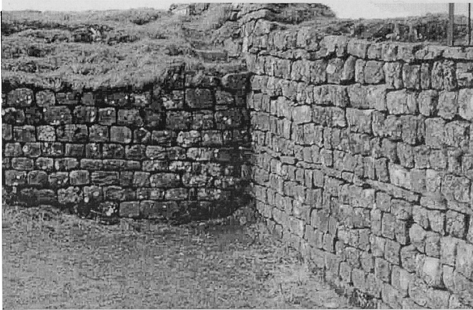
Plate 10 North wall of MC37, showing how irregularity of the stones makes precision of fixing unnecessary
