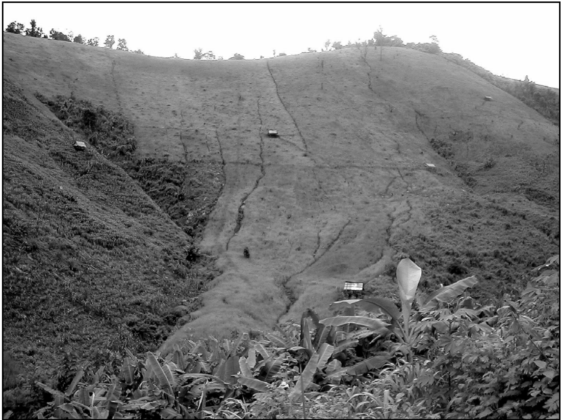
Photo 5.1: Linear erosion features on Ban Lak Sip land, July 2002
