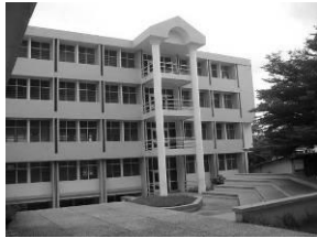
Fig.1: View of the building at CAP, KNUST
