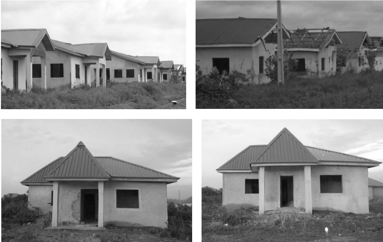
Fig 1: Prototype buildings in Minna showing variations of building components.
