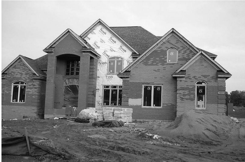
Fig 1: A mcmansion under construction.
