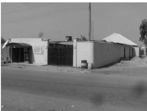
Figure 3: Constructed fence at Tunga Low cost Minna Source: Adedayo (2010a)
