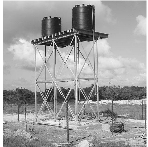
Pic 9: The Finished Water Tower. Source: Malaika Kids UK website.
