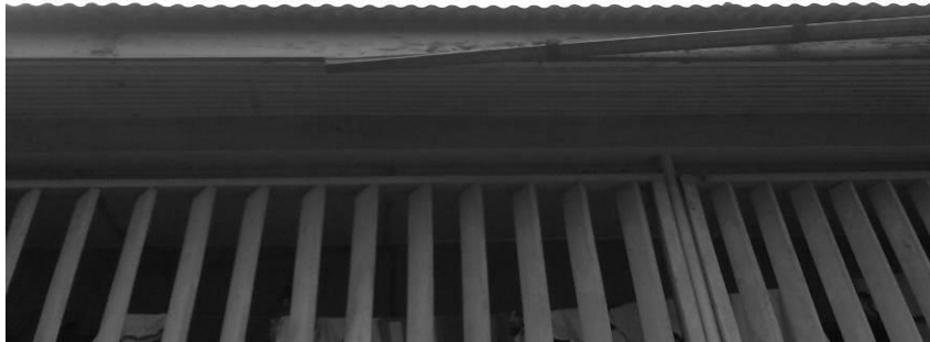
Fig 4: Showing local efforts at water harvestation from the roof.
