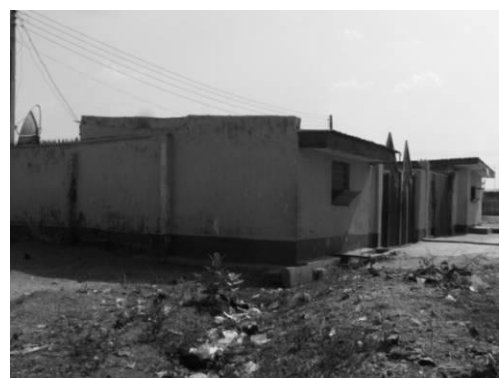
Figure 4: Constructed gate house at Tunga Low cost Source: Adedayo (2010a)
