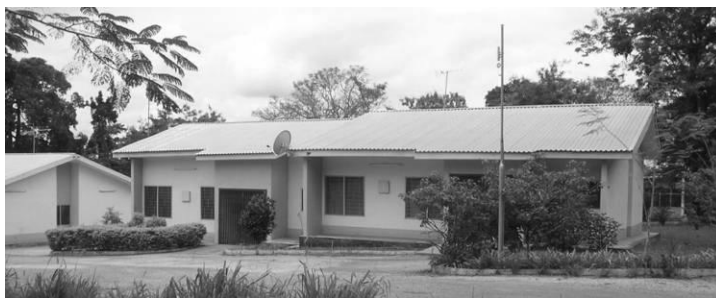
Fig.3: View of a semi-detached building, KNUST
