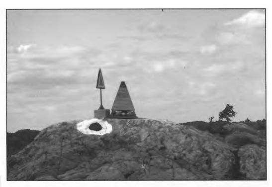
Finding your way through the rock-strewn North Channel, you must depend on aids to navigation. Shown here are three generations: a painted bulls-eye (well over 100 years old), a pyramid of wood held down by rocks, and a modern cement and steel triangle, destined to last 1000 years....
