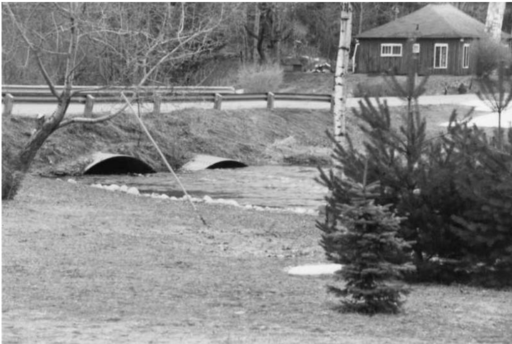
Photo 6. Milks Road crossing (from downstream) prior to restoration.
