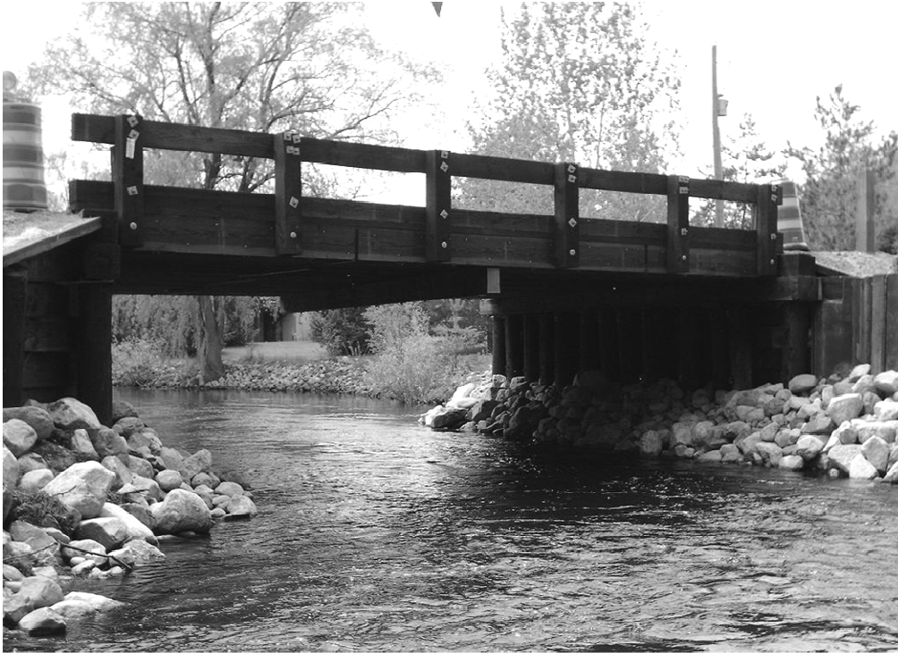
Photo 7. Milks Road crossing (from upstream) immediately following restoration.
