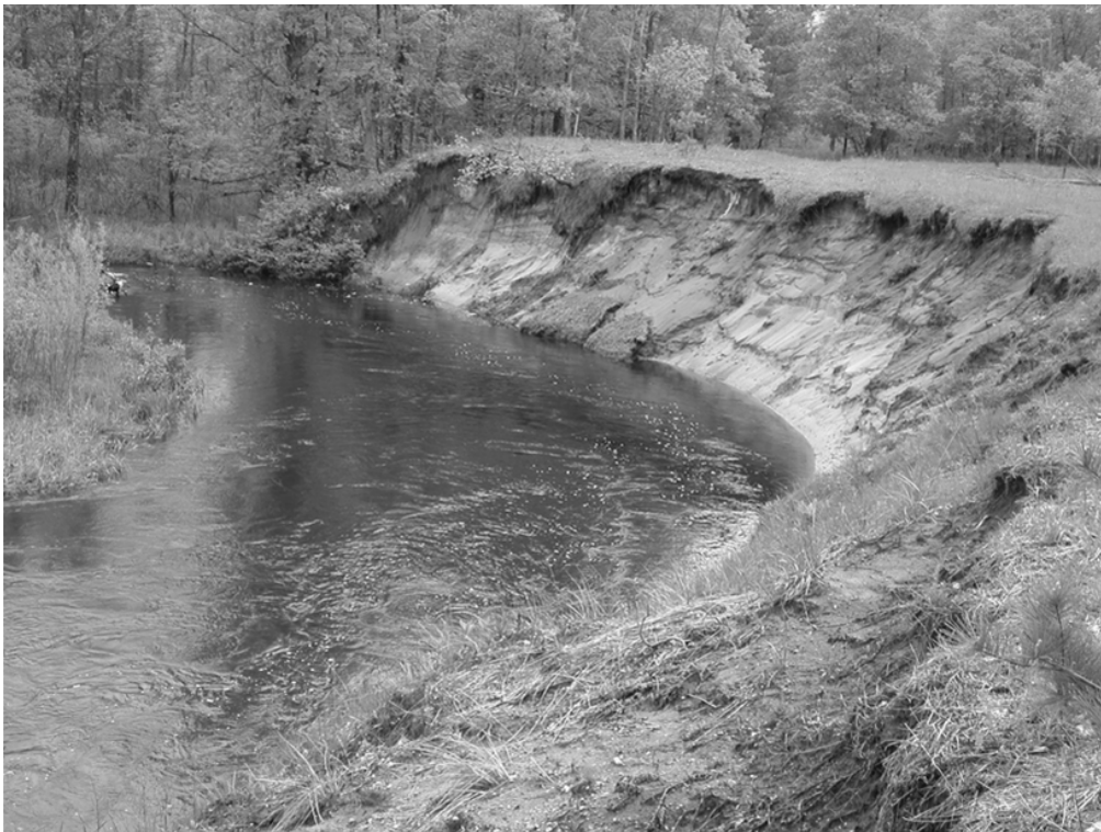
Photo 8. Upstream bank at Swain's Property prior to restoration.
