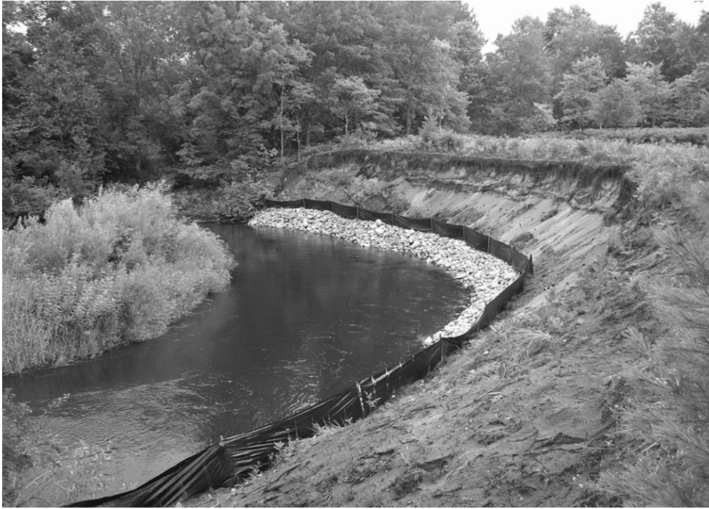
Photo 9. Upstream bank at Swain's Property immediately following restoration.
