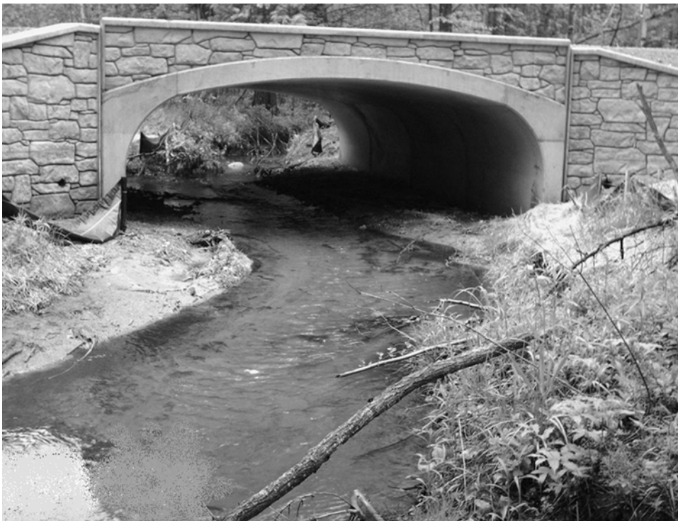
Photo 4. Sickie Creek immediately following restoration.
