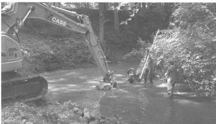
Heavy machinery was used to construct in-stream erosion controls in Sand Creek near Marne, Mich.
