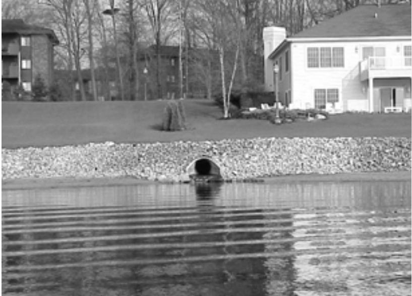
Unnatural shoreline of Mona Lake. Nonpoint source runoff from lawns and storm drains impairs lake water quality.
