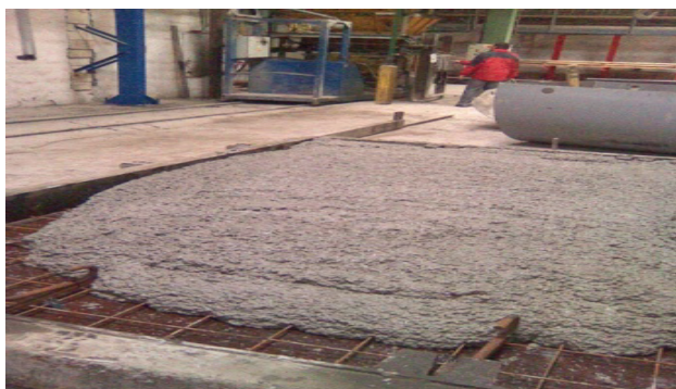
Figure 18 A view into the mould with reinforcement
