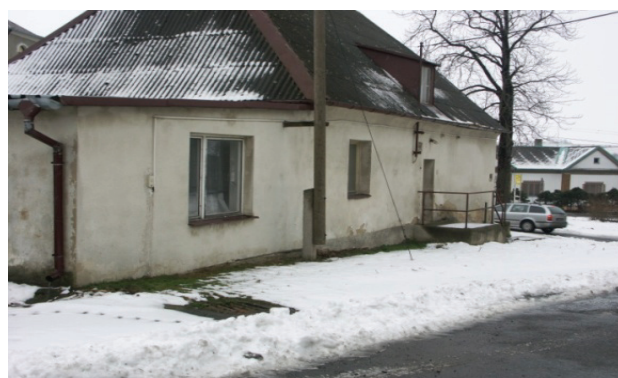
Figure 14 A view of reference building from the west before insulation by means of thermal insulating polyurethane mortar for rendering
