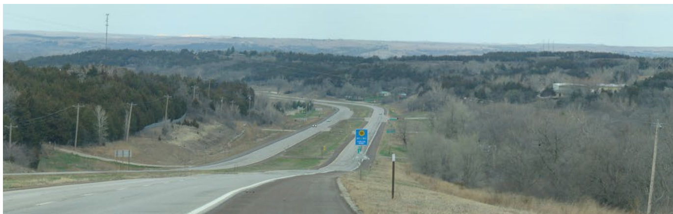
Figure 13. Panoramic view of the K-177 corridor
