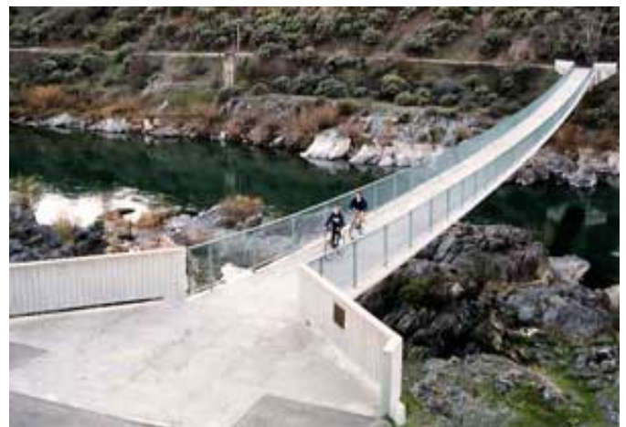
Figure 85. Concrete Stress Ribbon - Redding, California ( http://www.americantrails.org )
