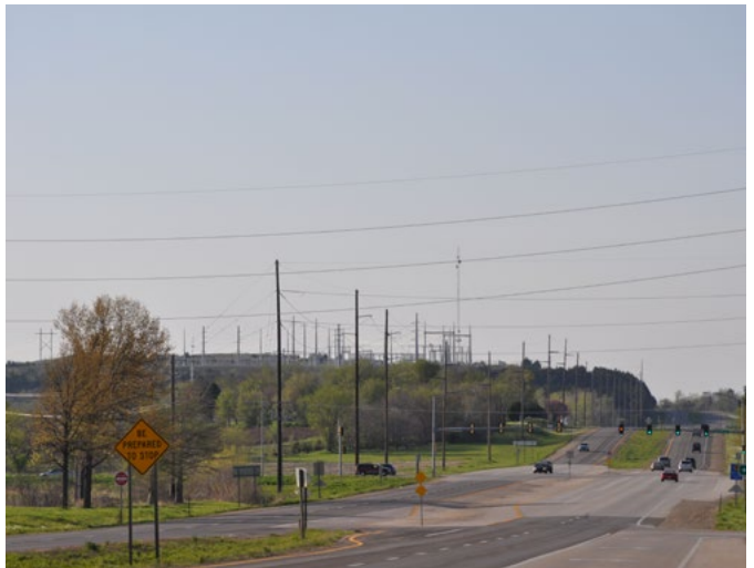
Figure 26. Kansas State University substation along Highway 24
