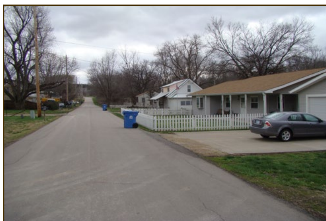
Figure 12. Residential development - Standel Road
