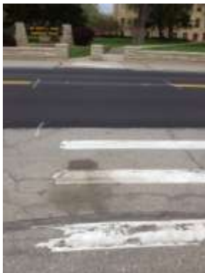
Figure 10. Crossing at Huebner Road.
