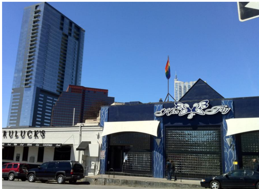
Figure 1: Kiss and Fly exterior façade
