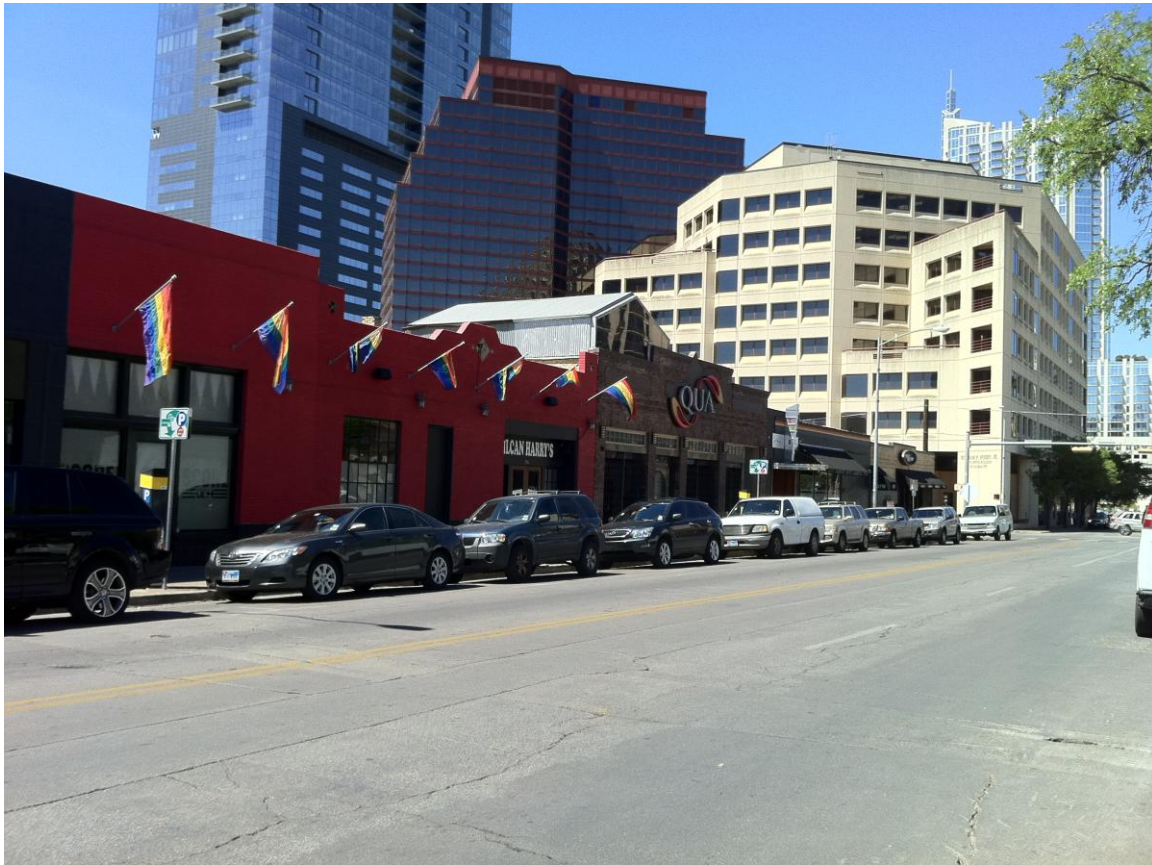
Figure 5: OCH on 4 th Street with W Hotel and state government building in background
