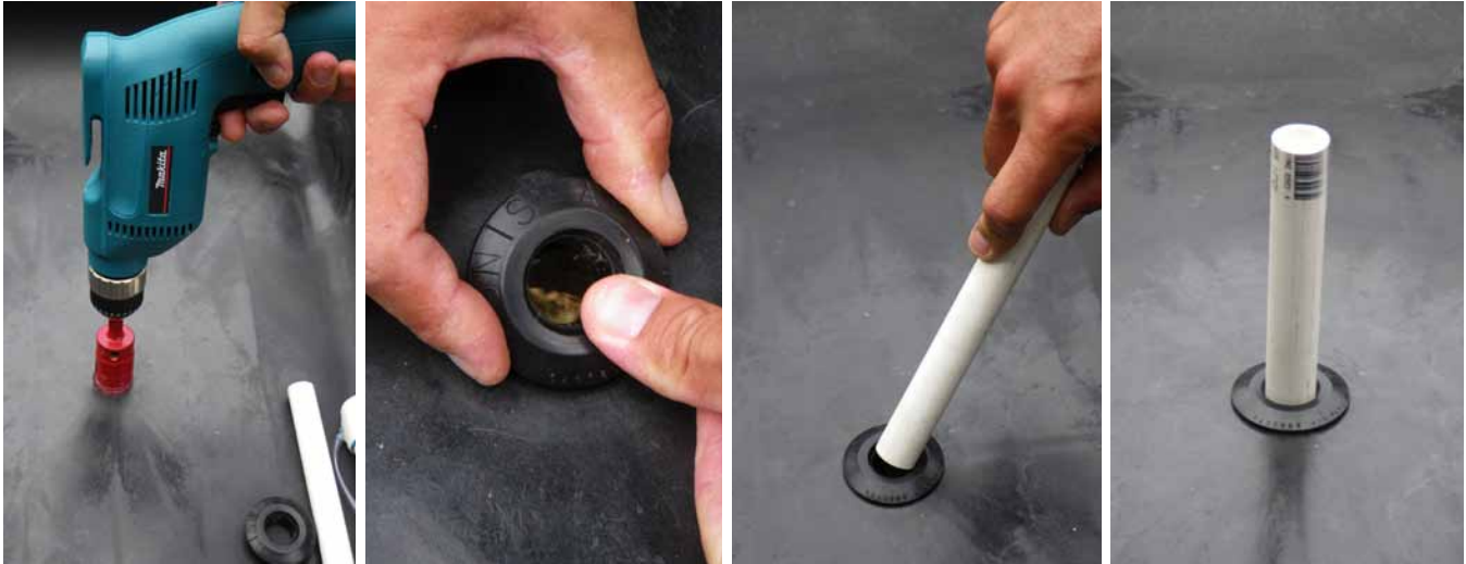
2. Installing a Uniseal fitting and standpipe in the grow-bed. Drill an appropriate size hole and insert the Uniseal in it; push the standpipe into the fitting and adjust the standpipe height to the desired level.
